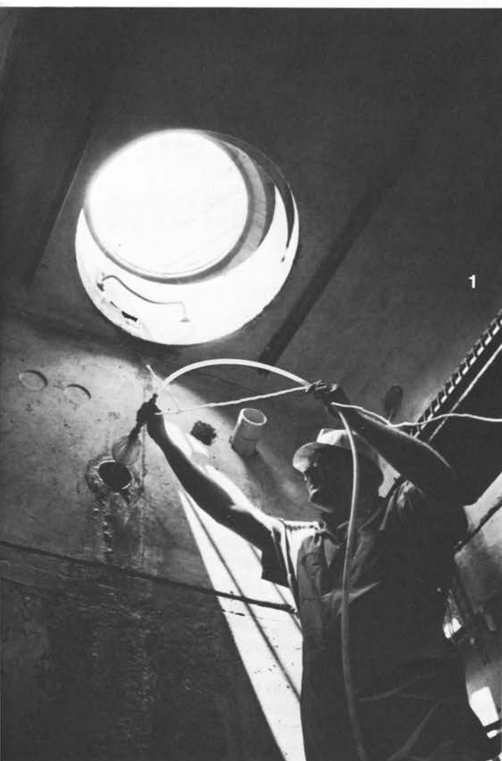
See-through. Chester people evaluate the performance of a "duct motor," a device that pulls a rodding line through a duct, the first step in installing cable in the duct. (1) Dave Gibson inserts the duct motor from a manhole. (2) Frank Fentzlaff (left) and Gibson observe the progress of the motor through a transparent duct,
