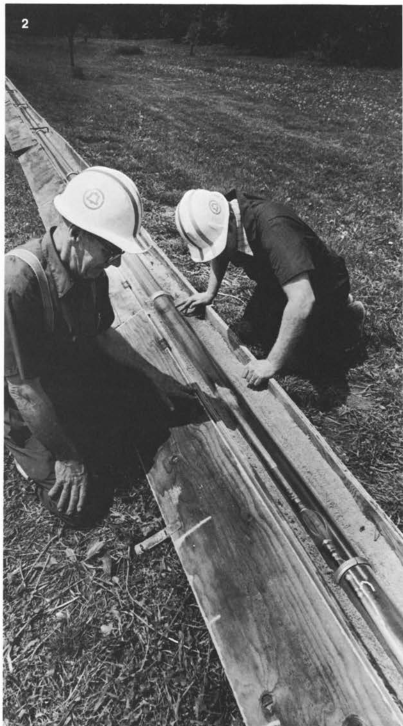
See-through. Chester people evaluate the performance of a "duct motor," a device that pulls a rodding line through a duct, the first step in installing cable in the duct. (1) Dave Gibson inserts the duct motor from a manhole. (2) Frank Fentzlaff (left) and Gibson observe the progress of the motor through a transparent duct,
