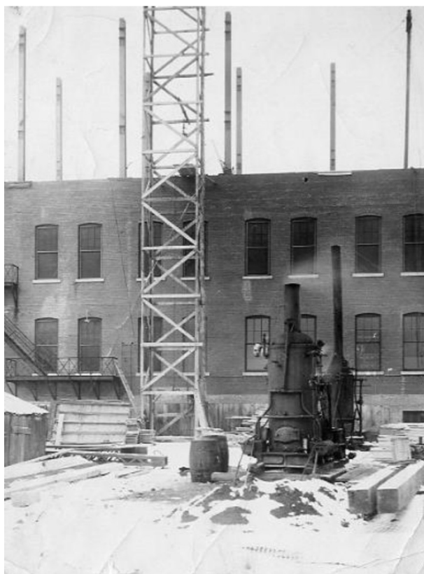
Grover exchange building under construction in 1923 (COURTESY BELL CANADA'S HISTORICAL COLLECTION)
