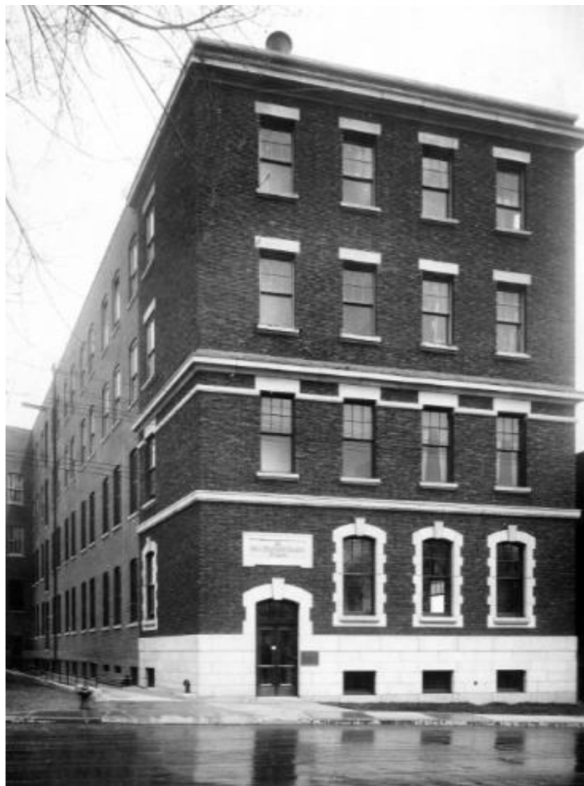
The Grover building with its 1925 two-story extension (photo taken in 1937)
