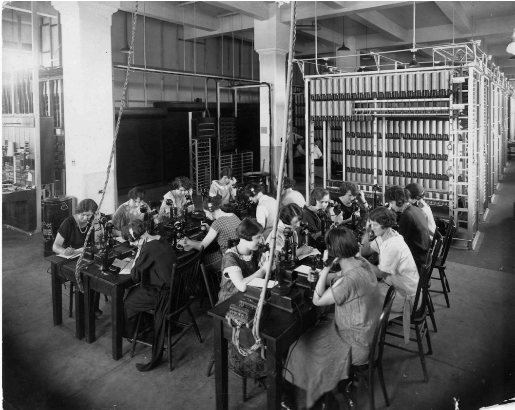
Ladies calling Grover subscribers just prior to cutover. New SXS equipment in background (COURTESY BELL CANADA'S HISTORICAL COLLECTION)
