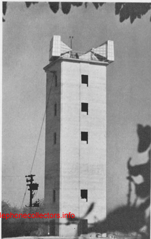
TD-2 repeater station at New Holland, Pa. The top floor houses the transmitting and receiving equipment which connects through waveguides to the antennas on the roof. Lower floors house rectifier, battery and power equipment.
