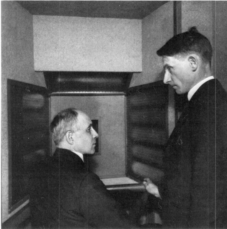
Fig. 3-2. F. B. Jewett, first president of Bell Laboratories (left), with F. Gray in the booth of the experimental television-telephone that permitted each person in a telephone conversation to see as well as hear the other.
