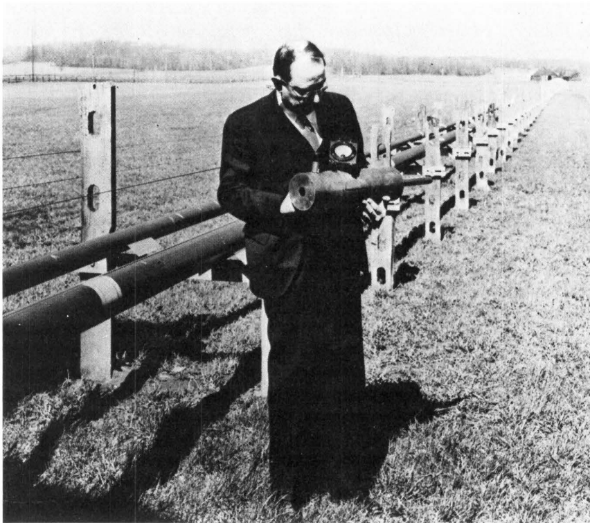
Fig. 6-1. G. C. Southworth in front of a TE_{01} waveguide transmission line built at Holmdel, New Jersey, in 1935. Southworth holds one of the resonant chambers used for tests of waveguide transmission.
