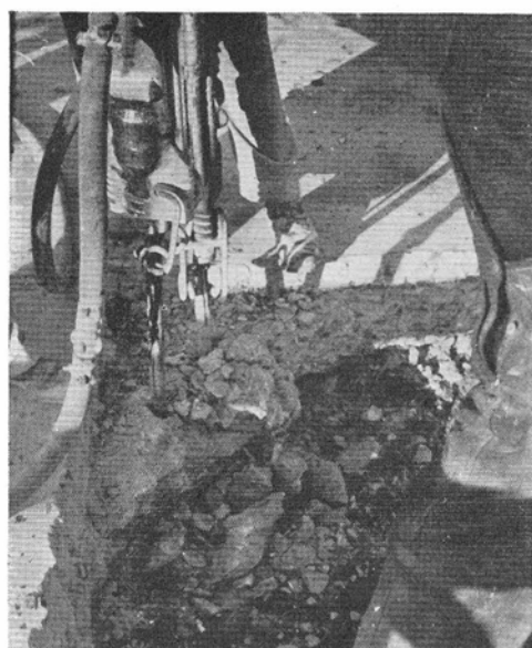
Breaking the concrete is some places 15" thick.
