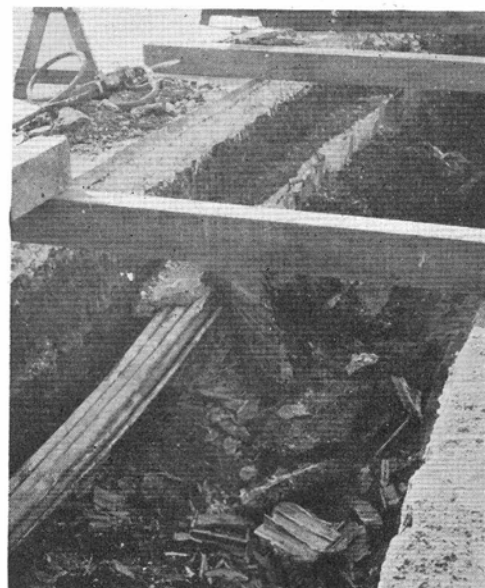
Breaking the tile and encasement preparatory to boxing the cables.
