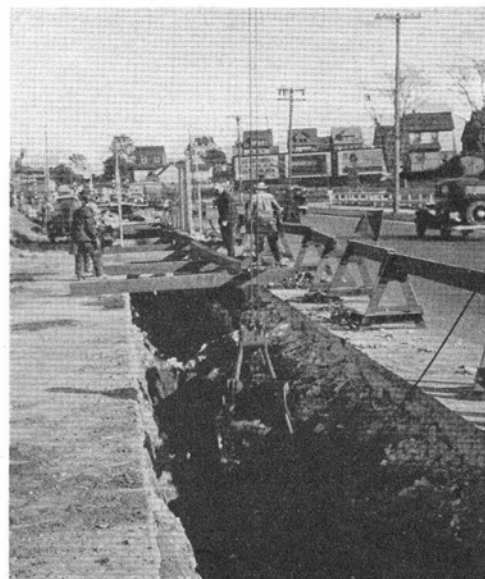
Excavating by use of Bay City Shovel. Used because of unusual depth required and to avoid relaying the dirt by hand on a series of platforms.
