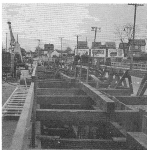
General view of job showing tight sheeting— heavy timbering, pumps, compressor and excavator.
