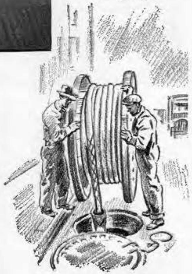
Now comes a cable with only two circuits, "coaxial cable," capable of carrying simultaneously 480 telephone conversations or 5,760 telegraph messages, and capable of transmitting images in motion—the future wire pathway for television. 55 miles of this new cable has been made by Western Electric and is now undergoing a trial between New York and Princeton, N. J.
