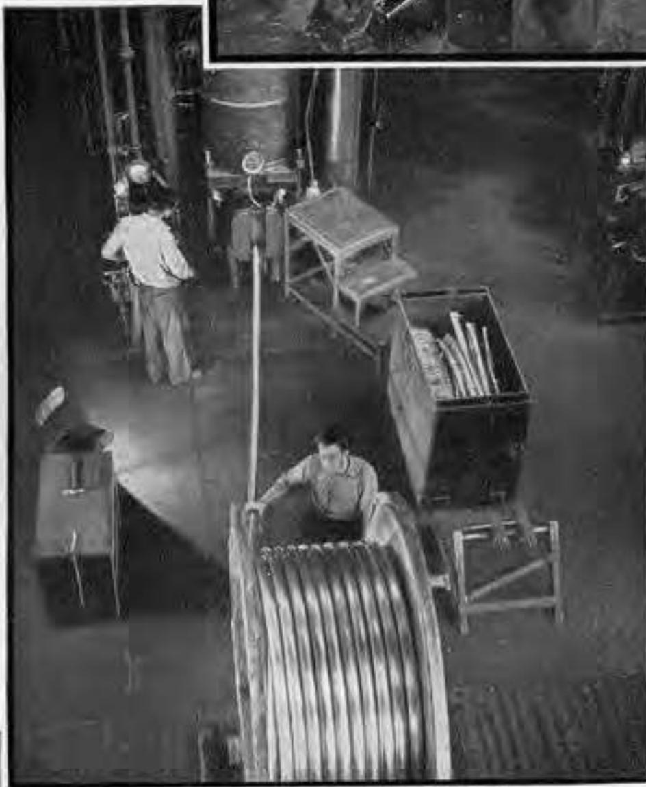
This lead press sheathes telephone cable with a lead antimony alloy.
