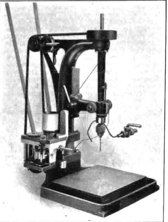
FIG. 3—TESTING MACHINE FOR SMALL DRILLS
