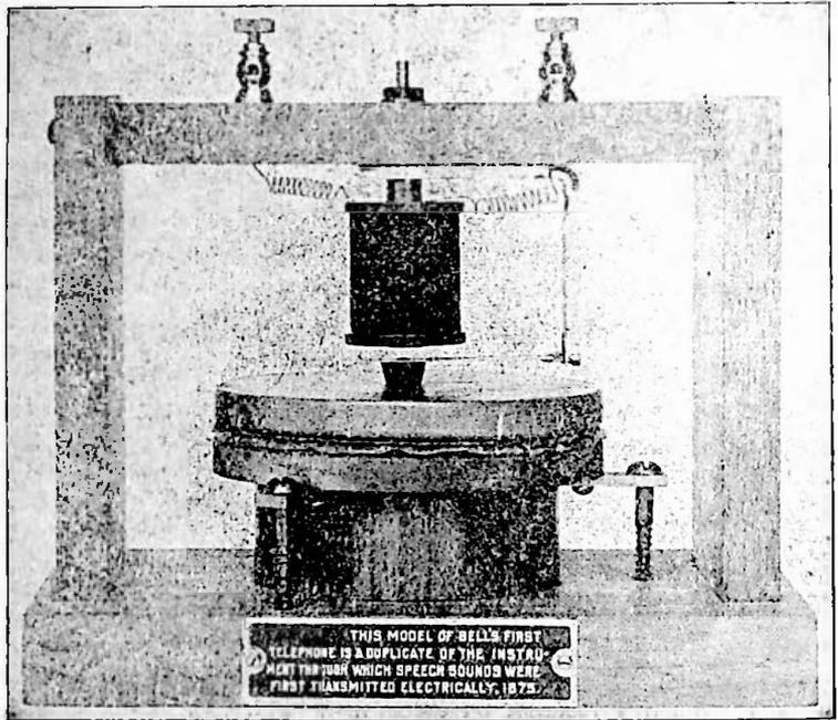
FIG. 8.—First electric speaking telephone. (Courtesy of Bell Telephone Laboratories.)
