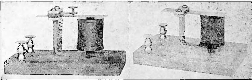
FIG. 7.—Bell's vibrating reed (transmitter left, receiver right). (Courtesy of Bell Telephone Laboratories.)
