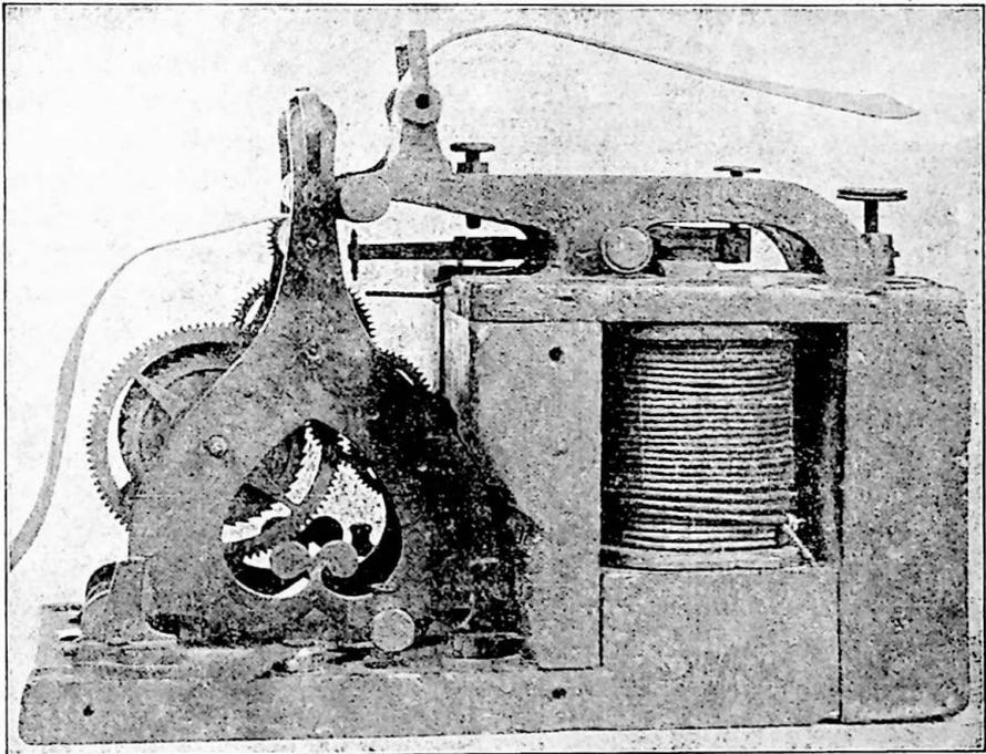
FIG. 3.—Original Morse telegraph recorder. (*Courtesy of Bell Telephone Laboratories.*)
