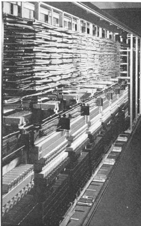
*Fig. 2—A rear view of the new board shows the compact grouping of the relays on their steel supporting structure and the accessibility of the multiple*
