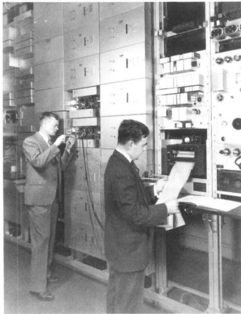
Fig. 15-1. Installation of A1 channel bank equipment at 32 Sixth Avenue, New York, 1938.
