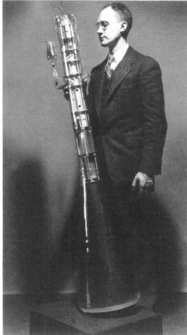
Fig. 6-19. The cathode-ray receiving tube used for the 1937 demonstration of television transmission over coaxial cable. The dimensions were chosen to obtain high linearity.
