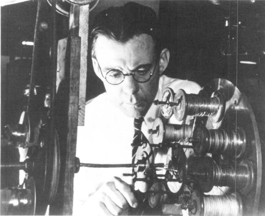
Fig. 6-6. J. F. Wentz making experimental coaxial conductors on an improvised stranding machine at Bell Laboratories.
