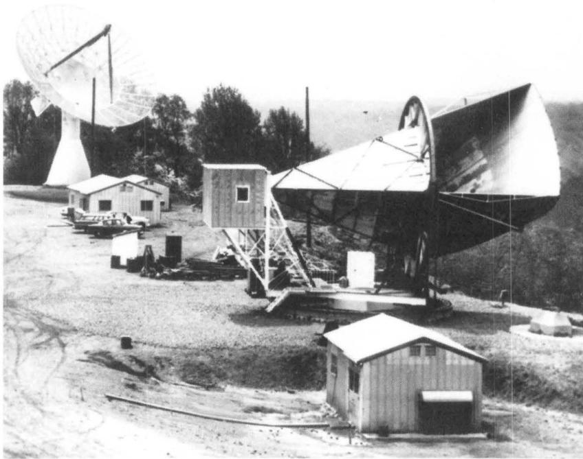
Fig. 13-3. The Crawford Hill antennas for Project Echo. *Right*, the horn-reflector antenna was the antenna later used by A. A. Penzias and R. W. Wilson to detect the 3°K background radiation from the origin of the universe.
