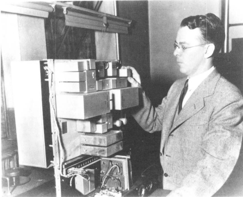
Fig. 4-1. H.S. Black holding one of the condensers from a negative-feedback amplifier being tested in 1930.
