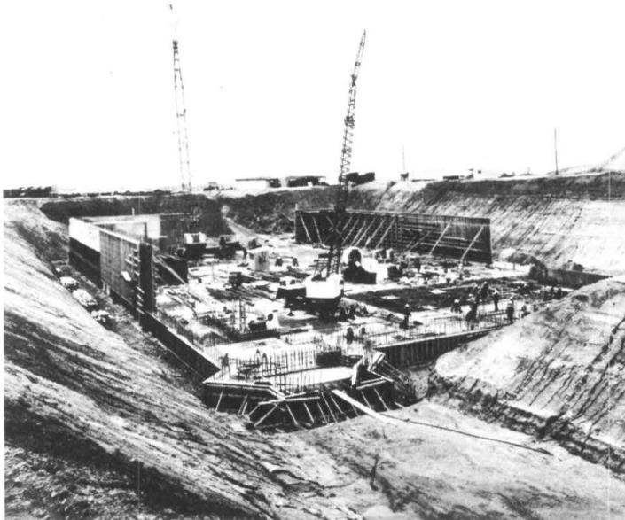
Fig. 10-10. One of the bomb-resistant main stations for the L4 coaxial system under construction on the Washington–Miami route, 1966.
