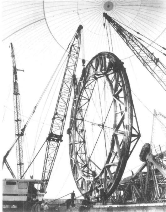
Fig. 13-11. Placing the 50-ton elevation wheel into position during construction of the Andover antenna.
