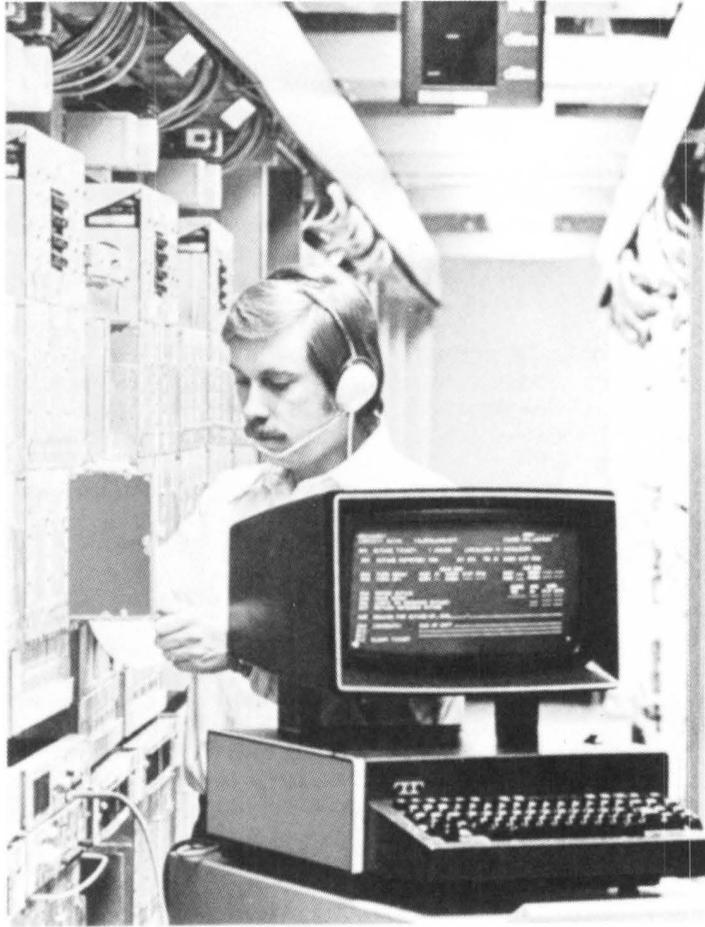
Fig. 23-15. A mobile CMS1A terminal in a transmission terminal equipment aisle of 4ESS switches.
