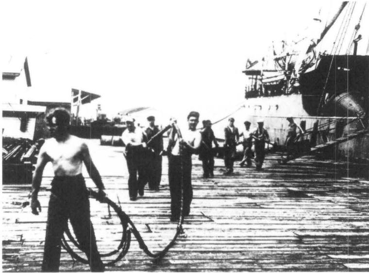
Fig. 12-3. The Key West–Havana submarine-cable repeater, 1950. The repeater appeared as a bulge on the cable three inches in diameter. With end tapers, it occupied about 35 feet of cable.
