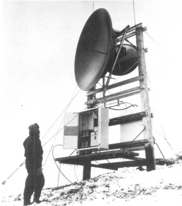
Fig. 11-19. The antennas and radio cabinets of a TL repeater on Chink's Peak, Idaho, one of the first installations of TL radio.
