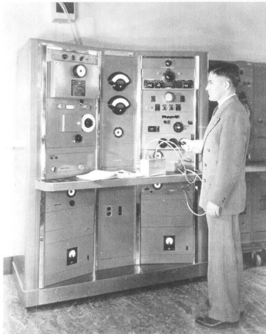
Fig. 8-7. Direct-reading phase and transmission measuring system, 1949.
