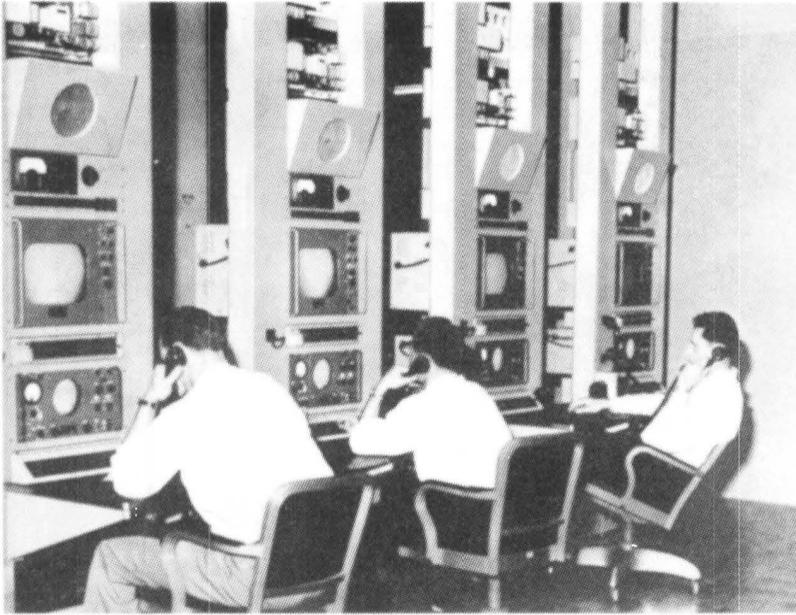
Fig. 22-9. Monitoring and test positions at a television operating center.
