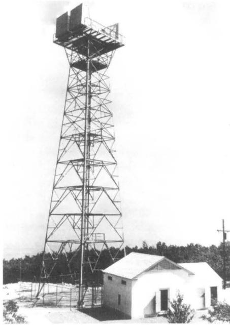
Fig. 11-8. A 125-foot steel tower for TD2.
