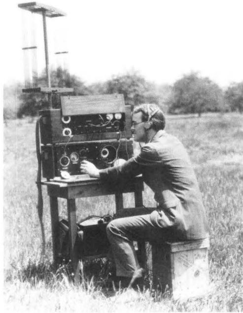
Fig. 3-1. Portable field-strength measuring equipment in use in the 1920s.
