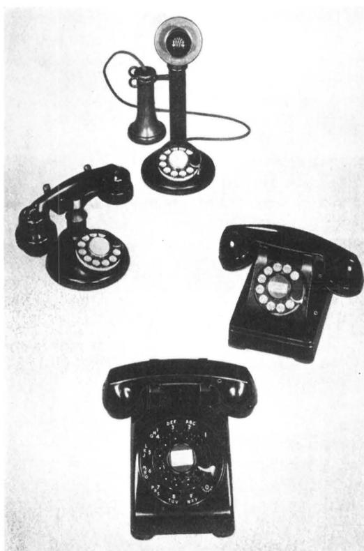
Fig. 22-2. The evolution of the telephone station set. *Top*, the candlestick deskstand of 1919; *left center*, the handset of 1927; *right center*, the 300 type combined set of 1937 (the ringer was included in the base); and, *bottom*, the 500 type set of 1950.
