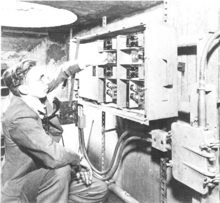
Fig. 6-16. The New York-Philadelphia trial amplifier. (a) Schematic of pilot-controlled regulating amplifier for experimental coaxial system. (b) Installed regulating amplifier in a manhole. The three-stage amplifier is made up of the vacuum tubes in the top compartment. The tubes in the lower section are part of the regulating network.
