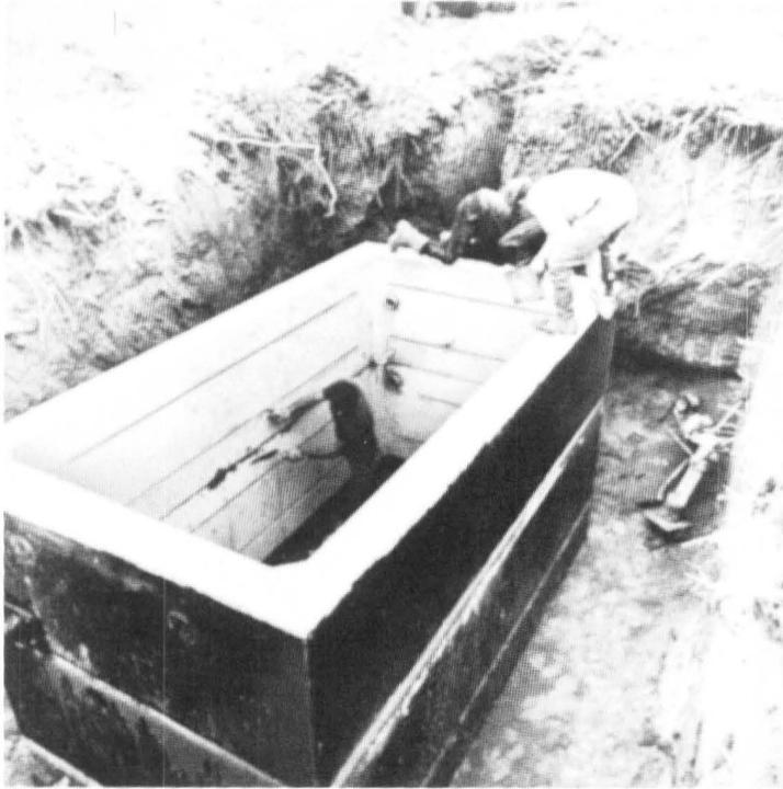
Fig. 10-27. A precast-concrete manhole of the type used to house L4 repeaters.
