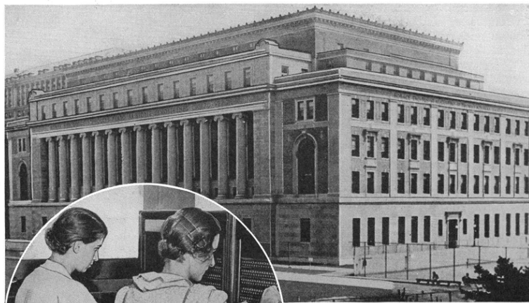
South Hall, Columbia University's new library. (Below) The telephone switchboard which is used in the delivery service of books to patrons of the reading rooms
