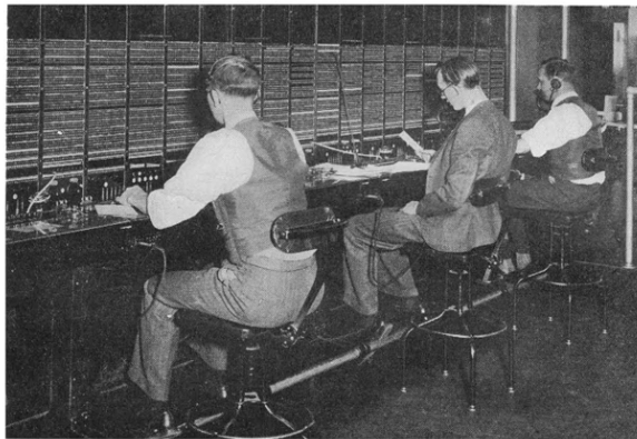
Circuit display board which keeps the Traffic Department advised of circuit conditions
