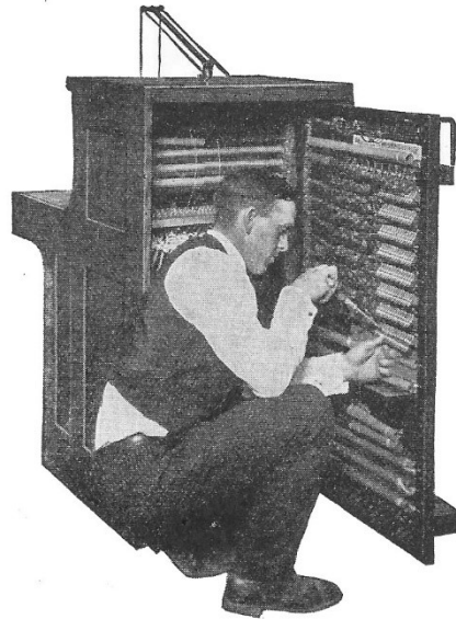
Installing the No. 2-A Trunk Circuit Plate on the No. 102 Switchboard
