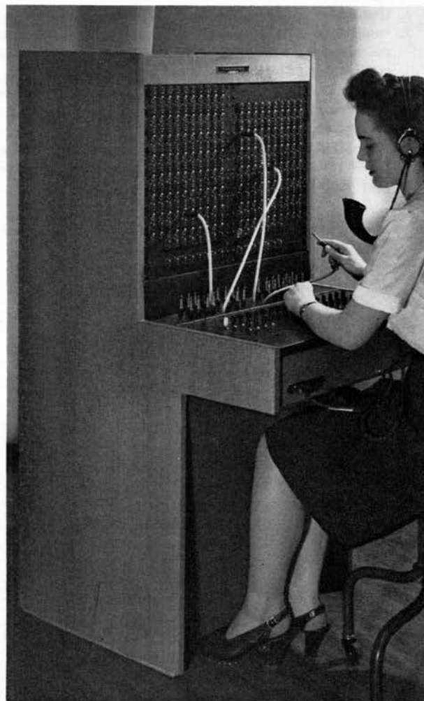
Typical Magneto Switchboard
