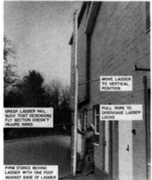
Fig. 25—Preparing to Lower Fly Section
