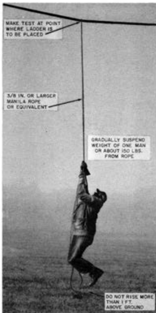
Fig. 2—Testing Strand Prior to Placing Ladder
