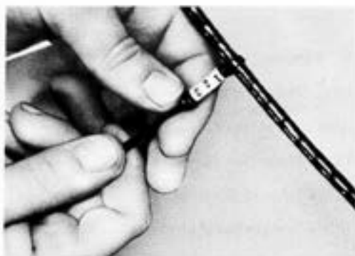
Fig. 2—♦Placing Tie and Marker♦
