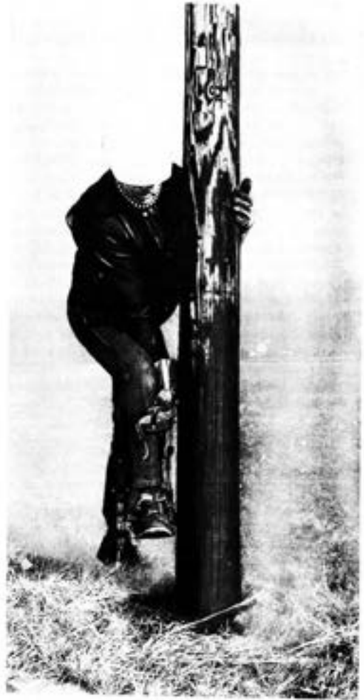
Fig. 15—Climber Holding
