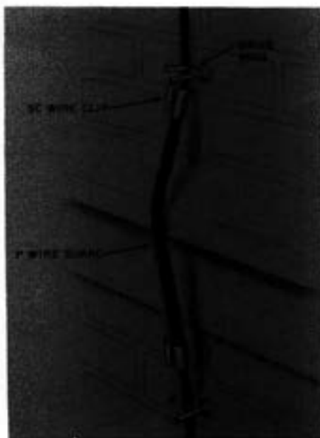
Fig. 3—Crossing Masonry Building Projection
