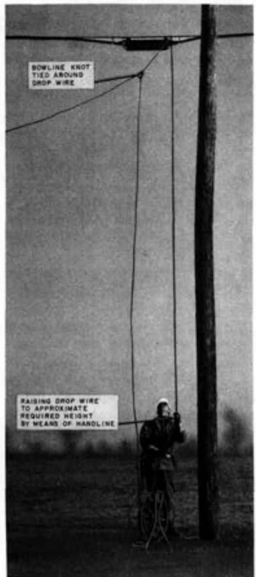
Fig. 5—Raising Drop Wire
