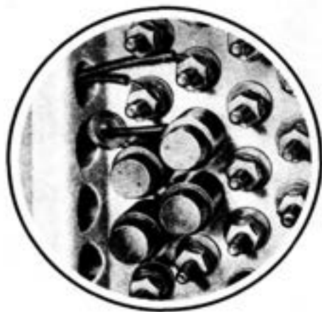
Fig. 19—Installed Binding Post Caps With KS-6660 Indicator
