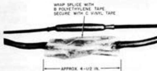
Fig. 23—Splice Wrapped With B Polyethylene Tape
