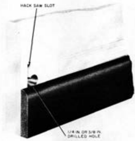
Fig. 15—Hole Through Wall for B Station Wire
