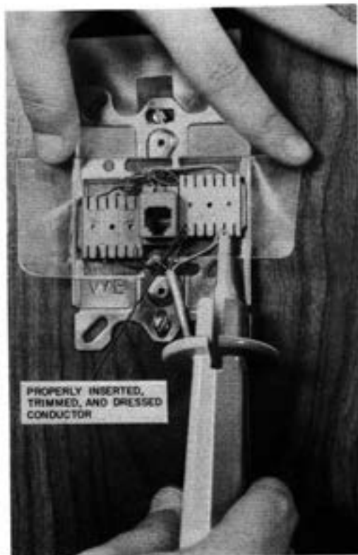
Fig. 12—Terminating Wire With Lead Insertion Tool in 630A4 Connecting Block
