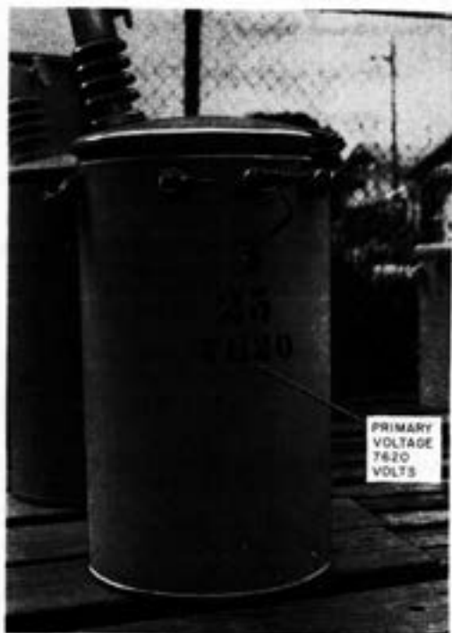
Fig. 9—Voltage Marking on Transformer
