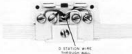
Fig. 6—Terminating Wire on No. 717 Terminal
