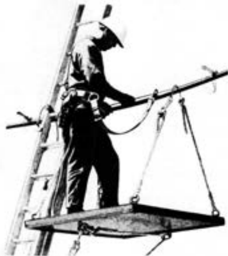
Fig. 8—Method of Using Safety Strap When Using Other Than a D, E, or F Belt
