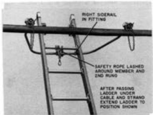
Fig. 46—E Ladder Support in Use
