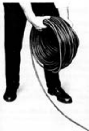
Fig. 2—Paying Out Cable
