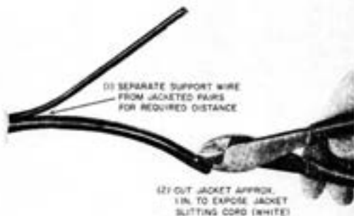
Fig. 14—Cutting Jacket With Diagonal Pliers
