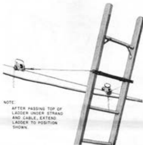
Fig. 42—D Ladder Support in Use
