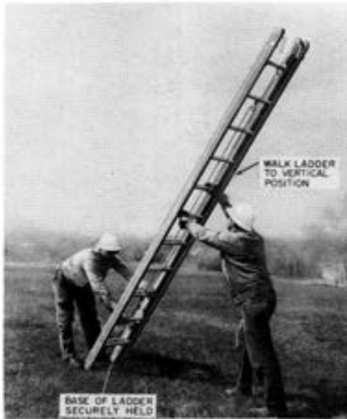
Fig. 27—Two Persons Raising Ladder
