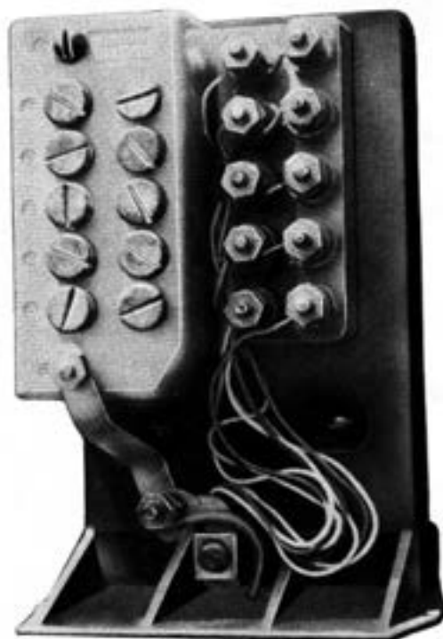
Fig. 23—142A1A Protector in C Customer Service Closure
