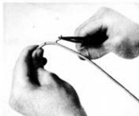
Fig. 8—Stripping D Station Wire
