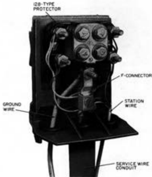
Fig. 28—Typical Protector Installation Using B Customer Service Closure
