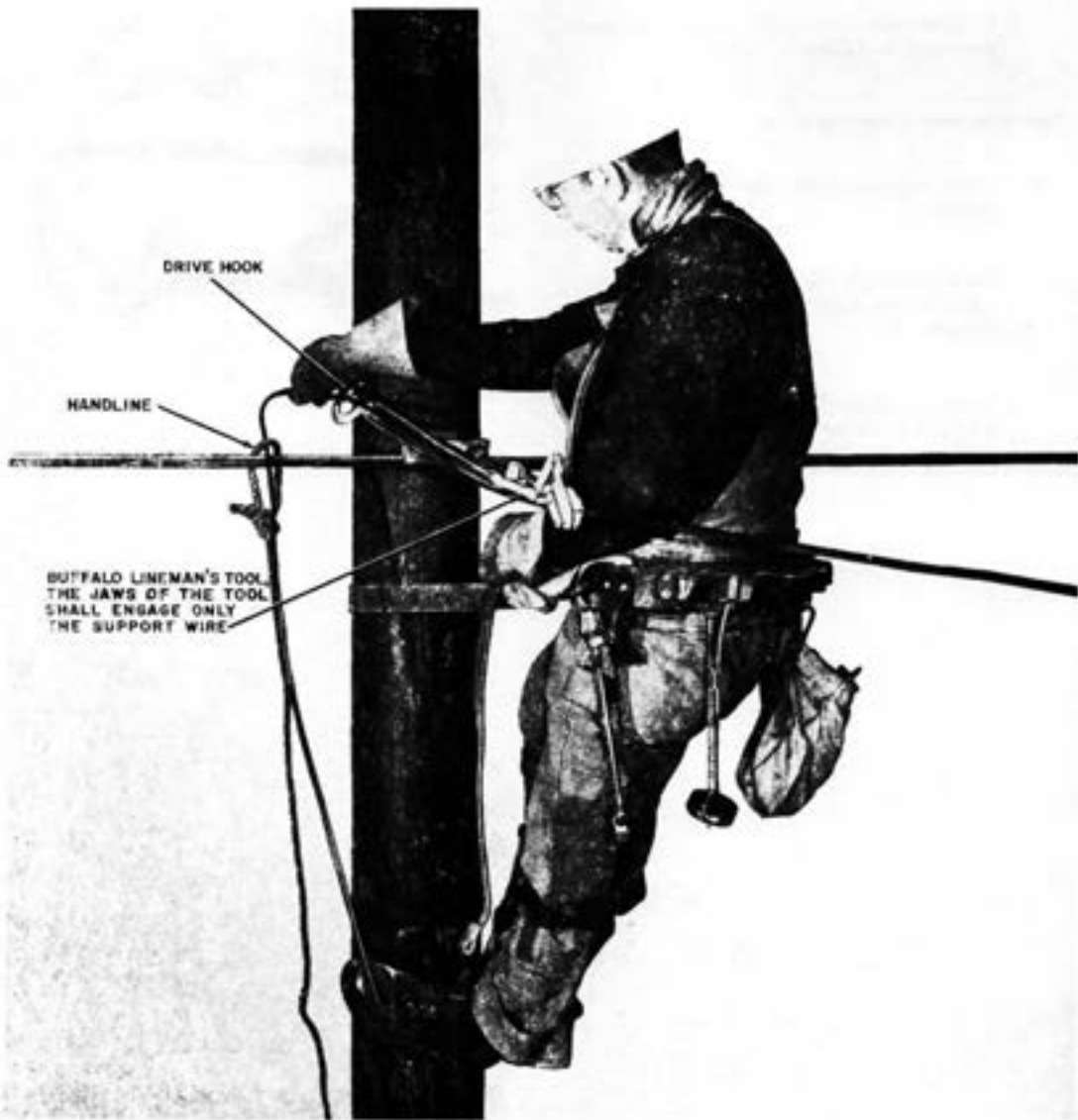
Fig. 9—Tensioning Wire With a Buffalo Lineman's Tool
