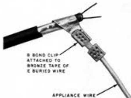
Fig. 27— Bonded Shield of E Buried Wire
