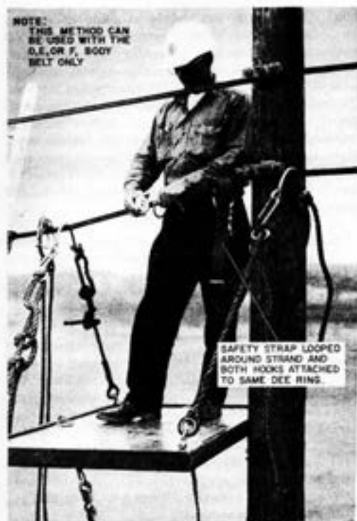
Fig. 7—Method of Using D, E, or F Body Belt With Safety Strap
