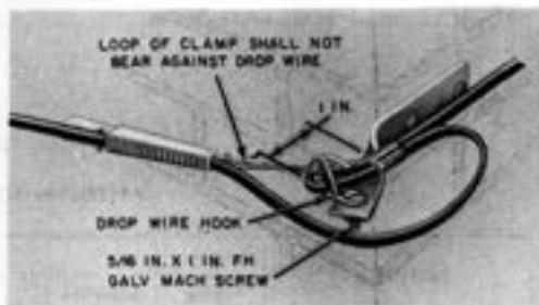
Fig. 7—First Attachment, Corner Bracket
