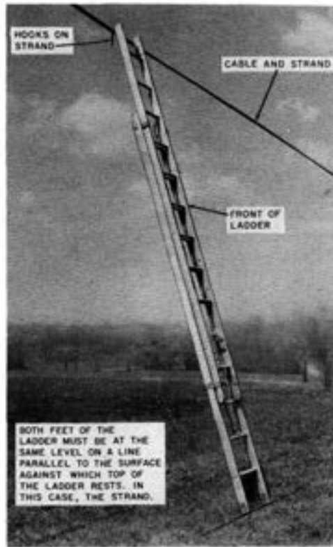
Fig. 12—Base of Ladder Properly Positioned
