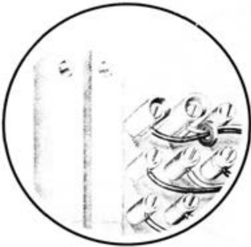
Fig. 27—Binding Post Insulators Installed at BD-Type Cable Terminals
