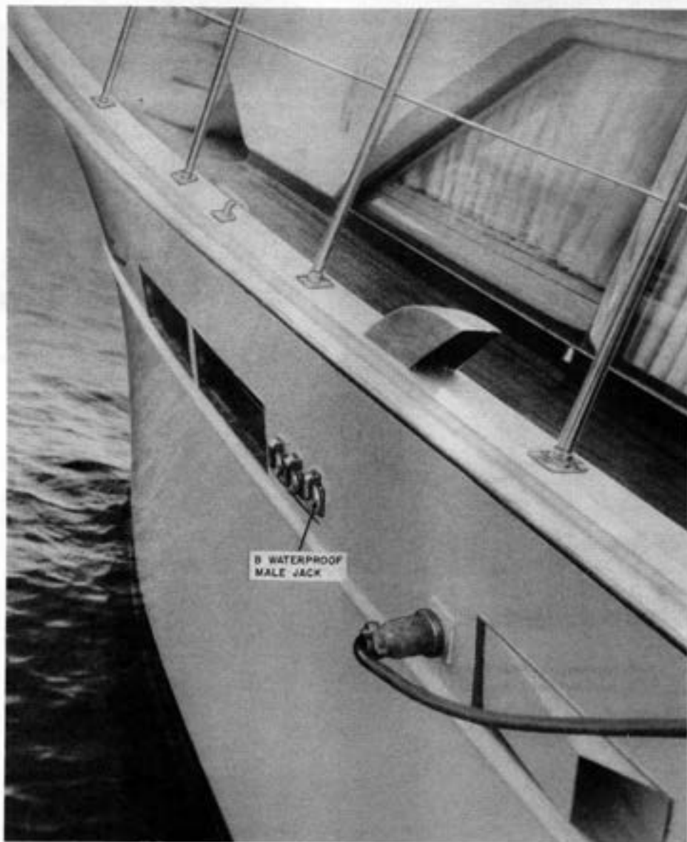
Fig. 22—Typical Outer Hull B Waterproof Male Jack Installation
