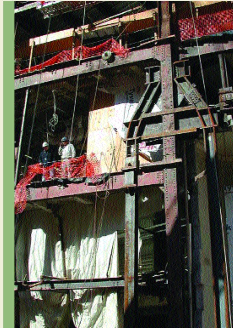
Entire column bays were destroyed as high up as the 13th story, and the East facade was decimated up to the 9th floor. Despite having two perimeter columns destroyed at their base, the sturdy building remained standing. However, falling debris damaged underground cable vaults and severed incoming Con Edison feeders, commercial steam service, domestic water mains and sewage piping.
