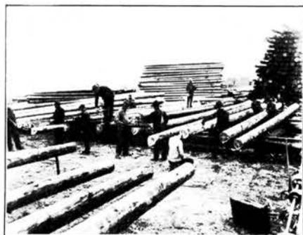
*Prospective telephone poles are carefully inspected in a concentration yard for any possible flaws.*
