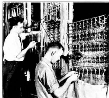
*On telephone equipment in the large central offices (exchanges) there are several million soldered joints containing lead.*
