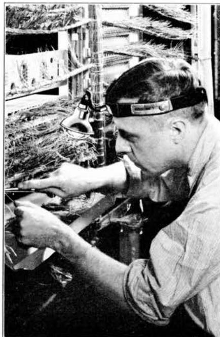
*This installer is connecting up the cotton and silk covered copper conductors in the telephone switchboard.*
