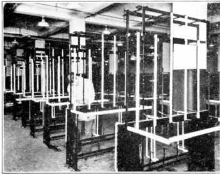
*Iron is used to make up much of the framework of the switchboard sections where thousands of telephone lines come together and where the called party is selected. Both the black and white framework sections shown above are of iron.*
