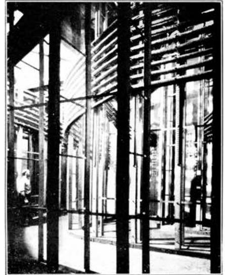
*A cable vault located far below a city street. Here is an orderly array of myriad telephone wires collected into cables and sheathed in coats of lead and antimony.*
