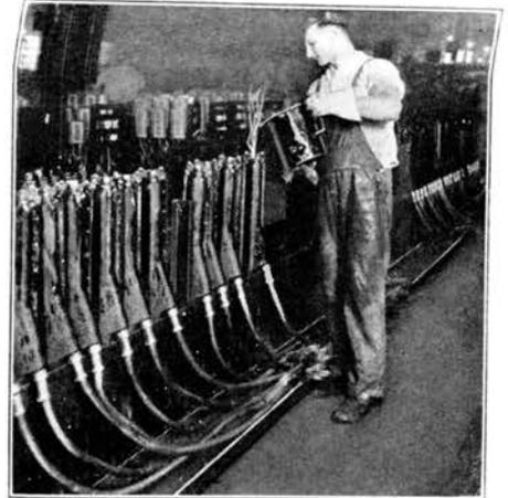
Asphalt in cable terminals, used when telephone wires are joined to a lead covered cable, prevents moisture working in among the wires.
