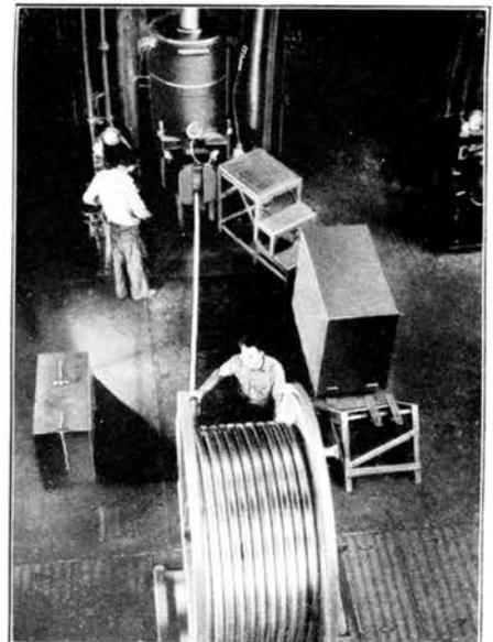
*Covering a cable with lead and antimony alloy sheath at the Point Breeze works of the Western Electric Company.*
