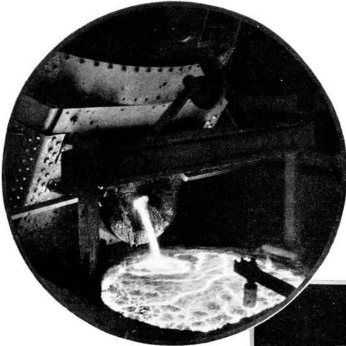
The tapping floor of a blast furnace, showing molten iron issuing from the furnace. Molten slag, being lighter than iron, floats on the top and is skimmed off, going down the trough at the right into a slag car. The molten iron flows off to the left into a hot-metal car.
