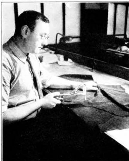
*Determining thickness of sueded leather used for base of telephone handsets.*
