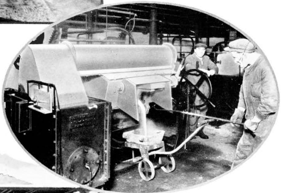
Below — Rod mills which break up the ore and classifiers used for fine grinding, in a South Dakota mine.
