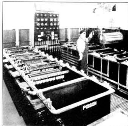
*Many parts of the telephone system are very delicate and must be protected against the effects of the atmosphere by plating.*
