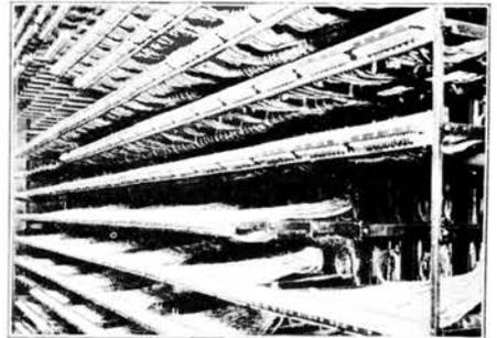
*Thousands of pounds of purified cotton and silk insulation, frequently impregnated with cellulose acetate lacquer, are used on the wires and cables in the telephone exchange to connect together the switchboards and auxiliary apparatus.*
