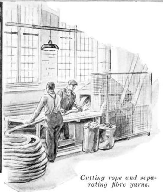
*Cutting rope and separating fibre yarns.*
