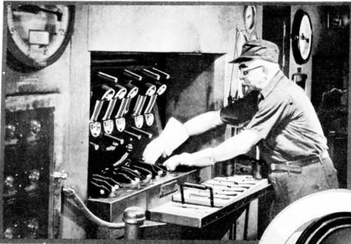
The powerful hydraulic presses for molding phenol plastic material take multiple dies so that as many as several dozen parts are made at once. Into each die the operator places either powdered plastic or pellets of plastic. The press is closed and in a very few minutes, the time depending on the size and type of the die, the jaws are opened and the parts, smooth surfaced as though hand-polished, emerge complete. The press at the left produces handset handles from powdered plastic.
