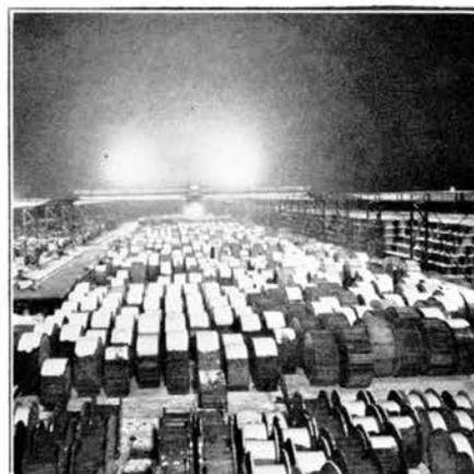
*In the yard of the world's largest telephone factory an overhead traveling crane picks up heavy reels of lead covered cable and carries them the length of the yard or across it in a very few minutes.*
