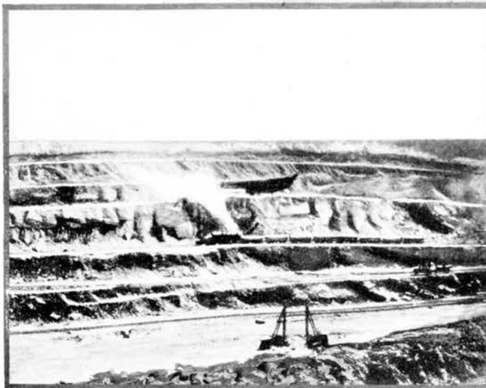
*In iron fields where the ore lies just under the surface, steam shovels scoop it up as the first step leading to the vessels which carry it through the Great Lakes to the important iron and steel manufacturing cities.*
