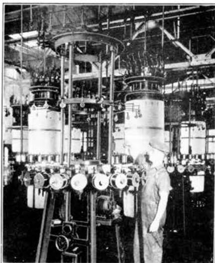
*Smaller, round ovens are used for baking varnish-like enamel on magnet type wire, some of which is finer than human hair. Wire passes from three to seven times through the troughs of enamel at the base of the machines and is finally taken up on spools held in frames like the one shown in the foreground.*
