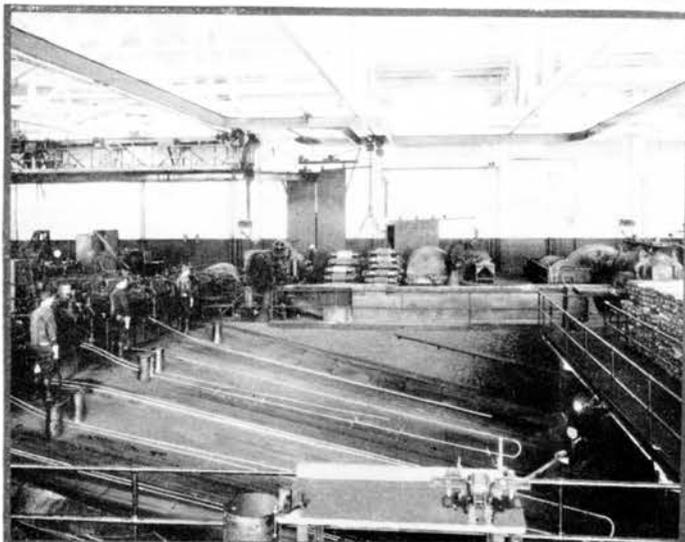
*Each pass of the bars through the rolls reduces the thickness of the copper and increases the length, so that now the bar, which was originally 54 inches long and 4 inches square, become a rod 1,200 feet long and only 1/4 inch in diameter.*
