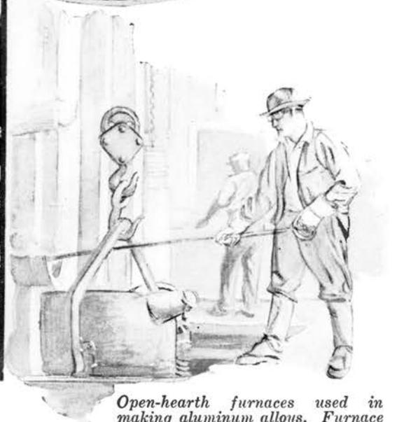
*Open-hearth furnaces used in making aluminum alloys. Furnace in the foreground is being tapped.*
