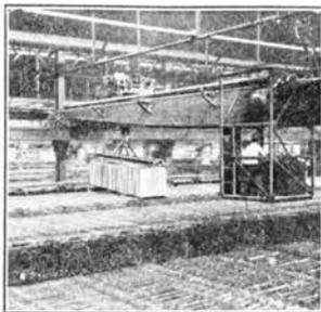
*In the electrolytic process used to produce practically pure copper, the copper is made into anodes which are put into a solution and an electric current gradually deposits it on plates of pure copper. The copper plates or cathodes when built up by deposits are more than 99% pure copper.*
