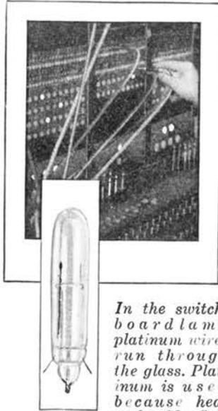
*In the switchboard lamp platinum wires run through the glass. Platinum is used because heat and cold affect it to about the same degree as glass and therefore the wires do not shrink away from the glass and let air into the lamps.*
