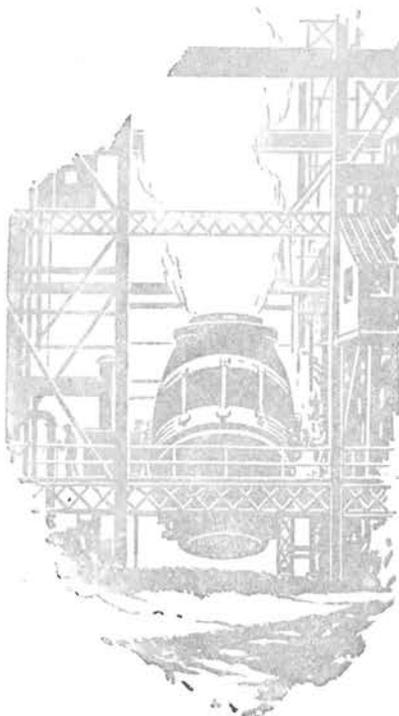
*A Bessemer Converter where tons of metal are handled at a time.*
