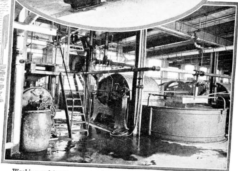
*Washing and beating rope to the proper dimensions for paper making.*
