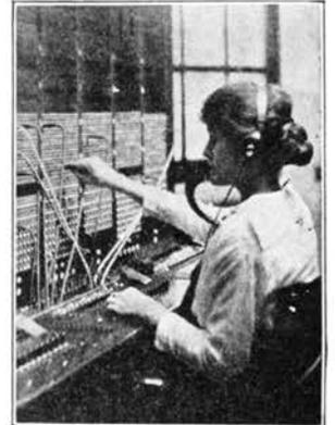
*When the switchboard is completed, the operator uses the silk and cotton covered voice pathways to bring to her ears the number wanted and to make a continuous path from one telephone user to the other.*
