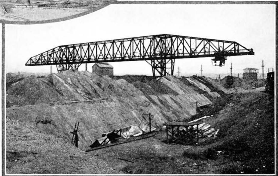
*A million ton storage yard for ore and coke and the ore bridge 507 feet long that picks up 14 tons of iron ore at each scoop of the shovel.*
