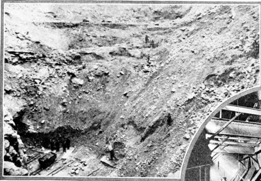
*Up in Ontario, Canada, where most of the world's nickel is mined the ore is dug from an open pit like this.*
