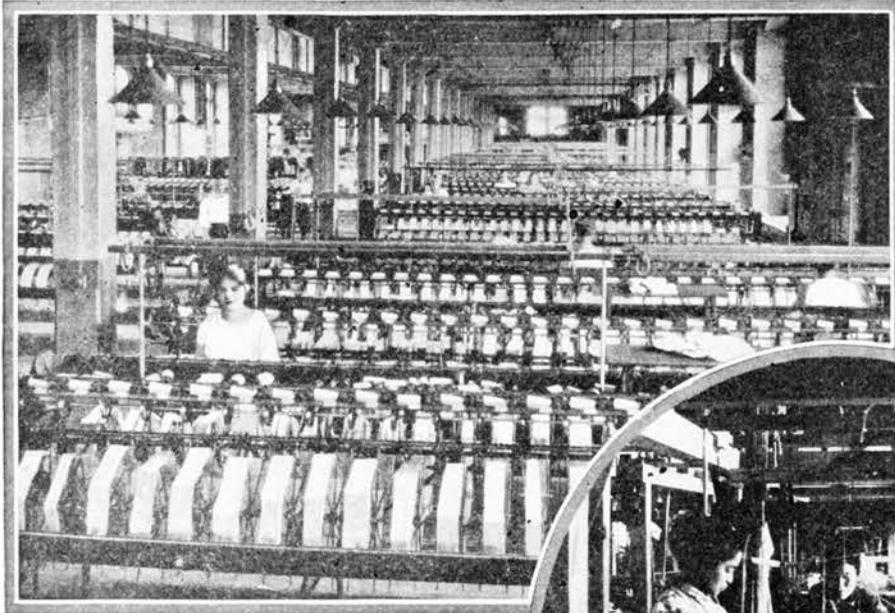
*Winding silk fibre from skeins on to bobbins in an American silk mill.*
