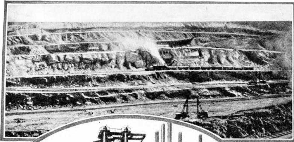
*In iron fields where the ore lies just under the surface, steam shovels scoop it up as the first step leading to the vessels which carry it through the Great Lakes to the great iron and steel manufacturing cities.*
