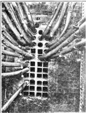
*Under the streets from manhole to manhole the lead covered cable carrying hundreds of pairs of wires lies in clay conduit, either square or round.*
