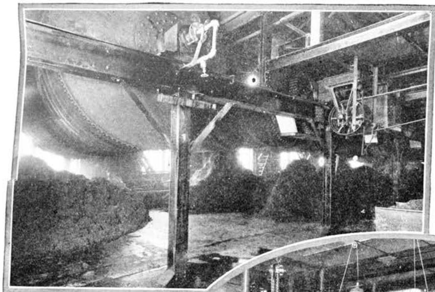
*Below—The dry end of a paper making machine where paper is dried, calendered and rolled.*
