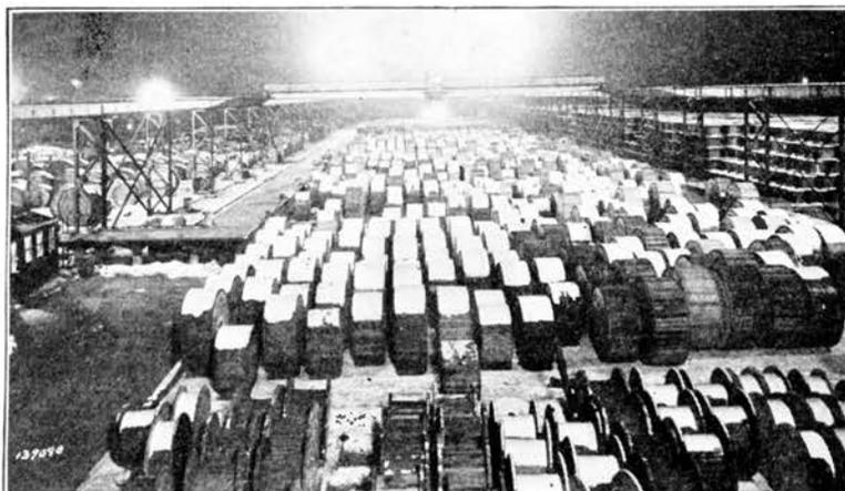
*In the yard of the world's largest telephone factory this overhead traveling crane picks up heavy reels of lead covered cable and carries them the length of the yard or across it in a very few minutes.*
