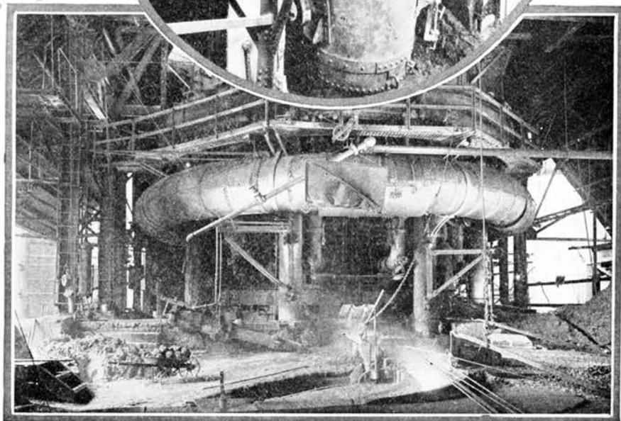
*After the metal has been melted out of the ore, the furnace is "tapped" and the molten iron drawn off.*
