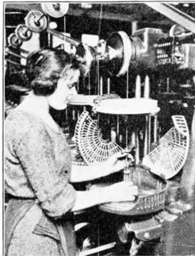
*A strip of insulating paper is wrapped around each copper wire for lead covered cable. Different colors identify the wires. In the closeup the wire is seen coming up through the center of the flat roll of paper while the bobbin spins around it, wrapping the paper on in a long spiral.*
