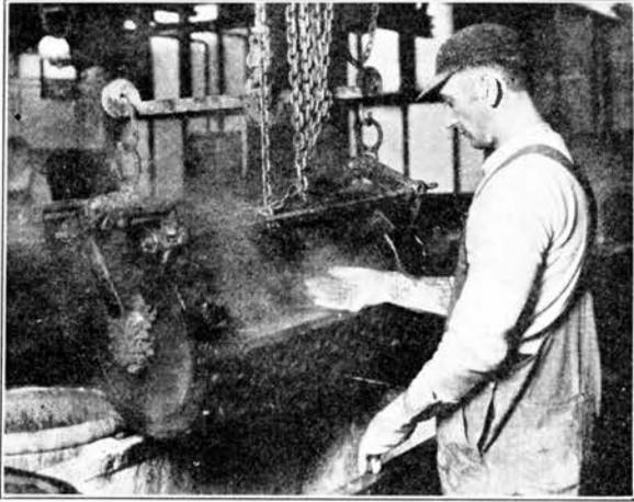
*Galvanizing, a process that protects iron from moisture and rust, is done by immersing the parts to be coated in molten zinc.*
