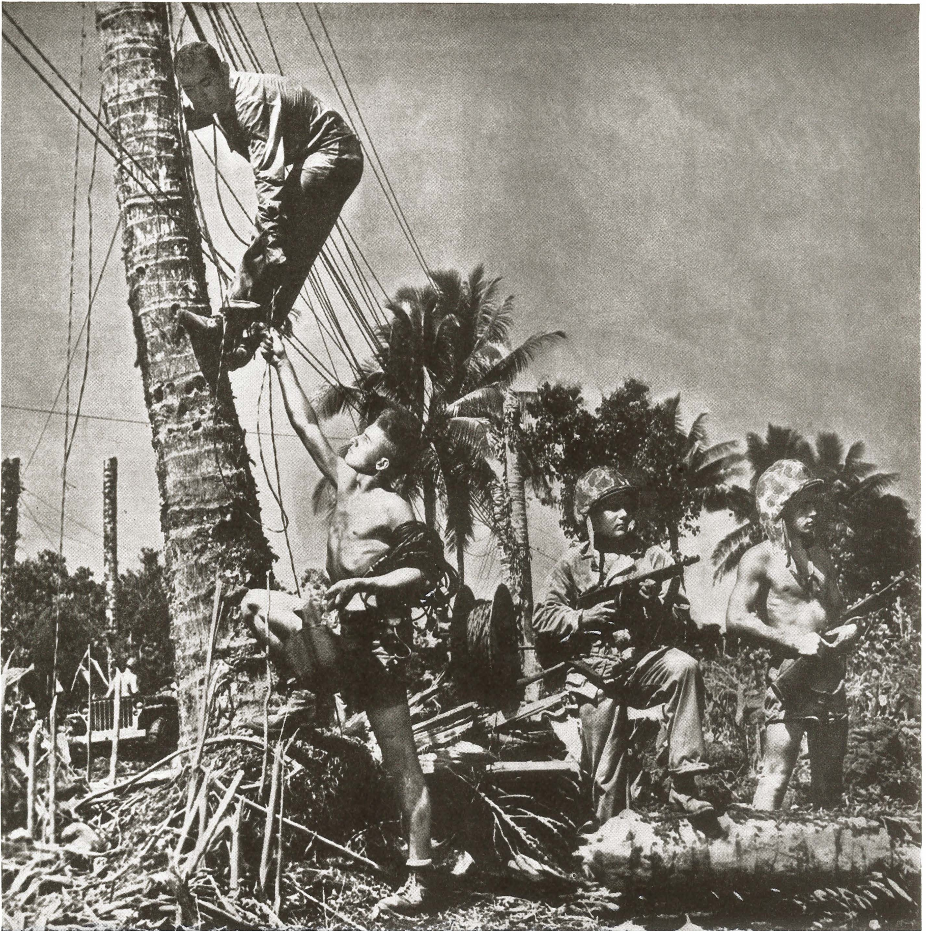
U. S. MARINES ON BOUGAINVILLE use palm trees for telephone poles as they string communication lines. Two stand guard with carbine and sub-machine gun, as protection against snipers.
