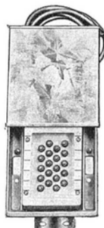
“F” Type Cable Terminal (Open)
