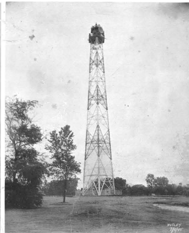
This tall tower at Nutley, part of a radio link between Nutley, Telegraph Hill and the I. T. & T. Building in New York, is triangular in shape. Except for bolts and steel gusset plates, the structure is of pre-fabricated timber
