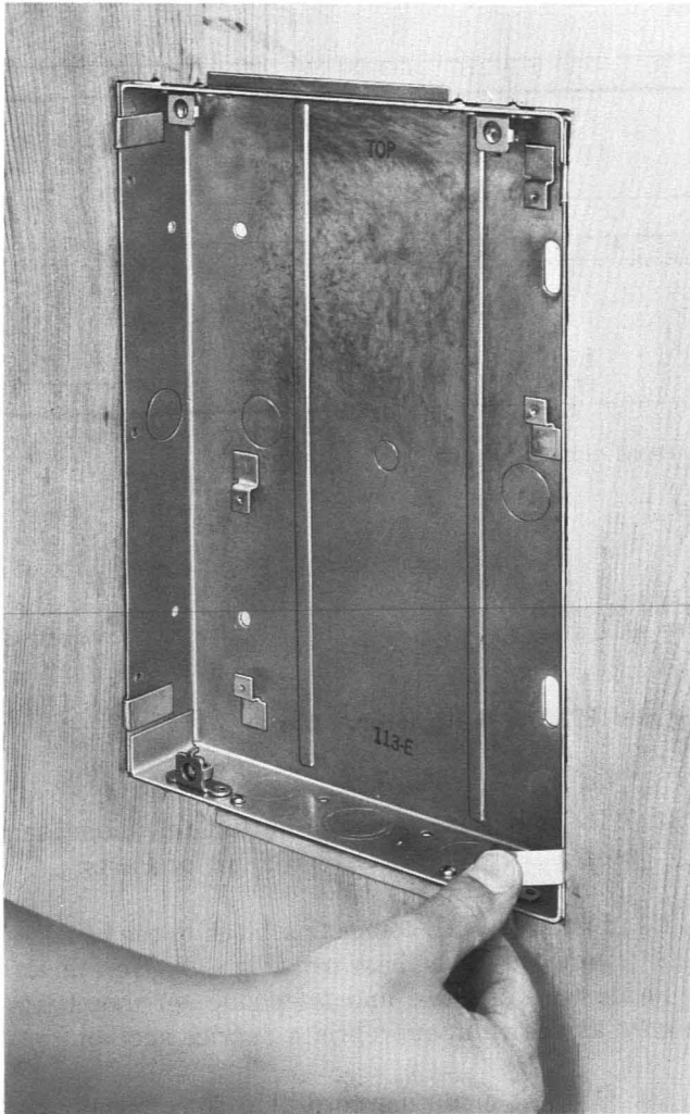
Fig. 6—113E Apparatus Box with D-179941 Kit of Parts Installed
