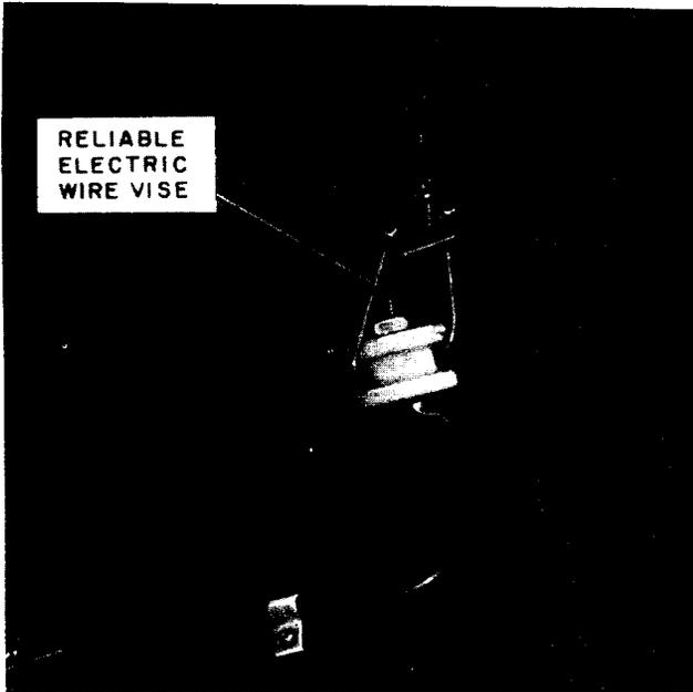
**Fig. 4—F Coaxial Wire Attached to First House Attachment With a Reliable Steel Wire Vise**
