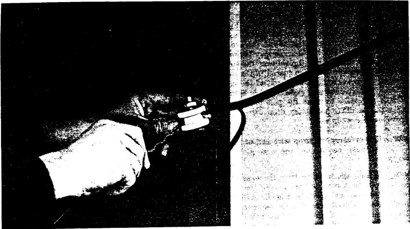
Fig. 3—Attaching F Coaxial Wire to First House Attachment With Preformed Deadend
