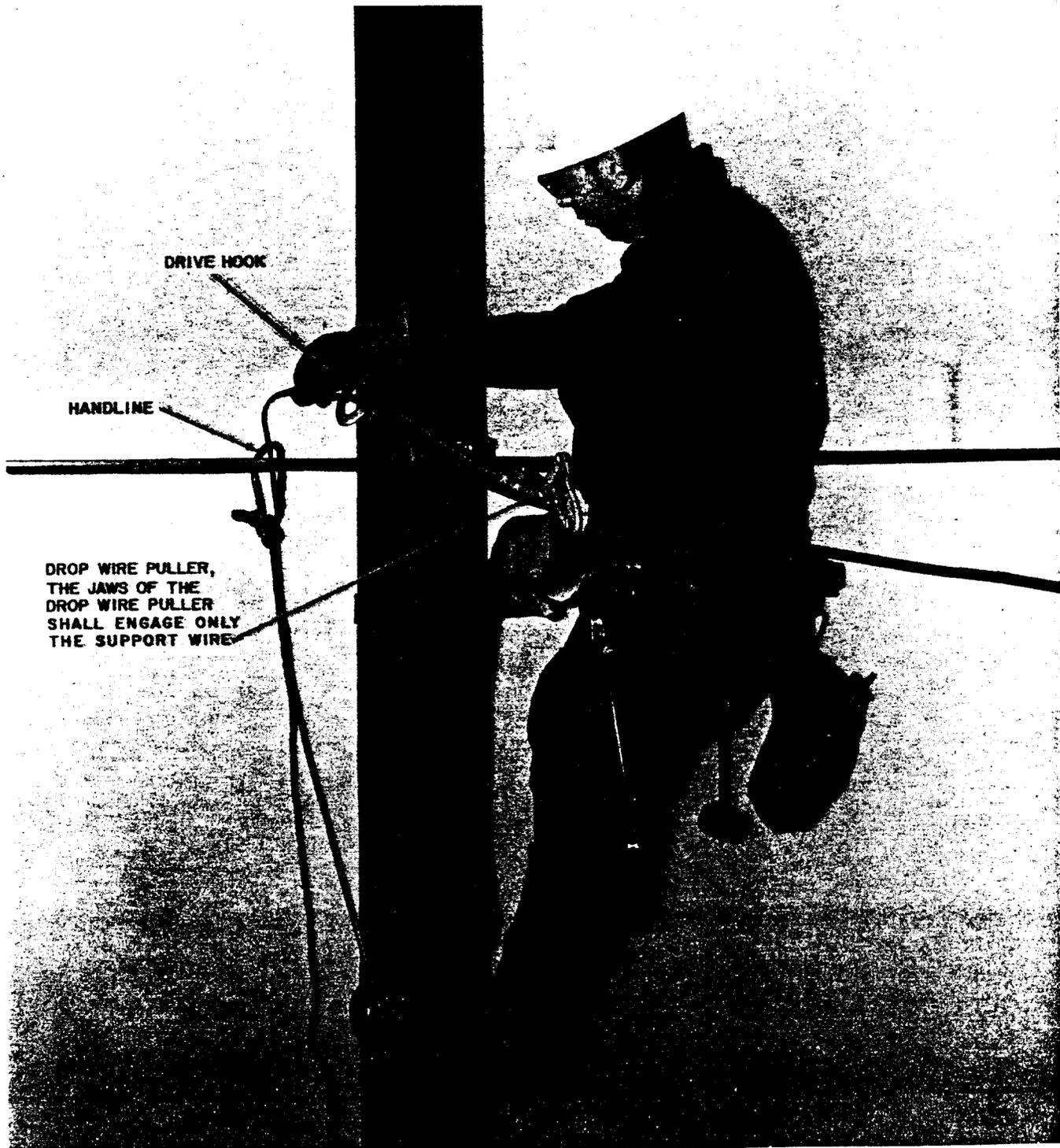
Fig. 8—Installed Drop Wire Puller
