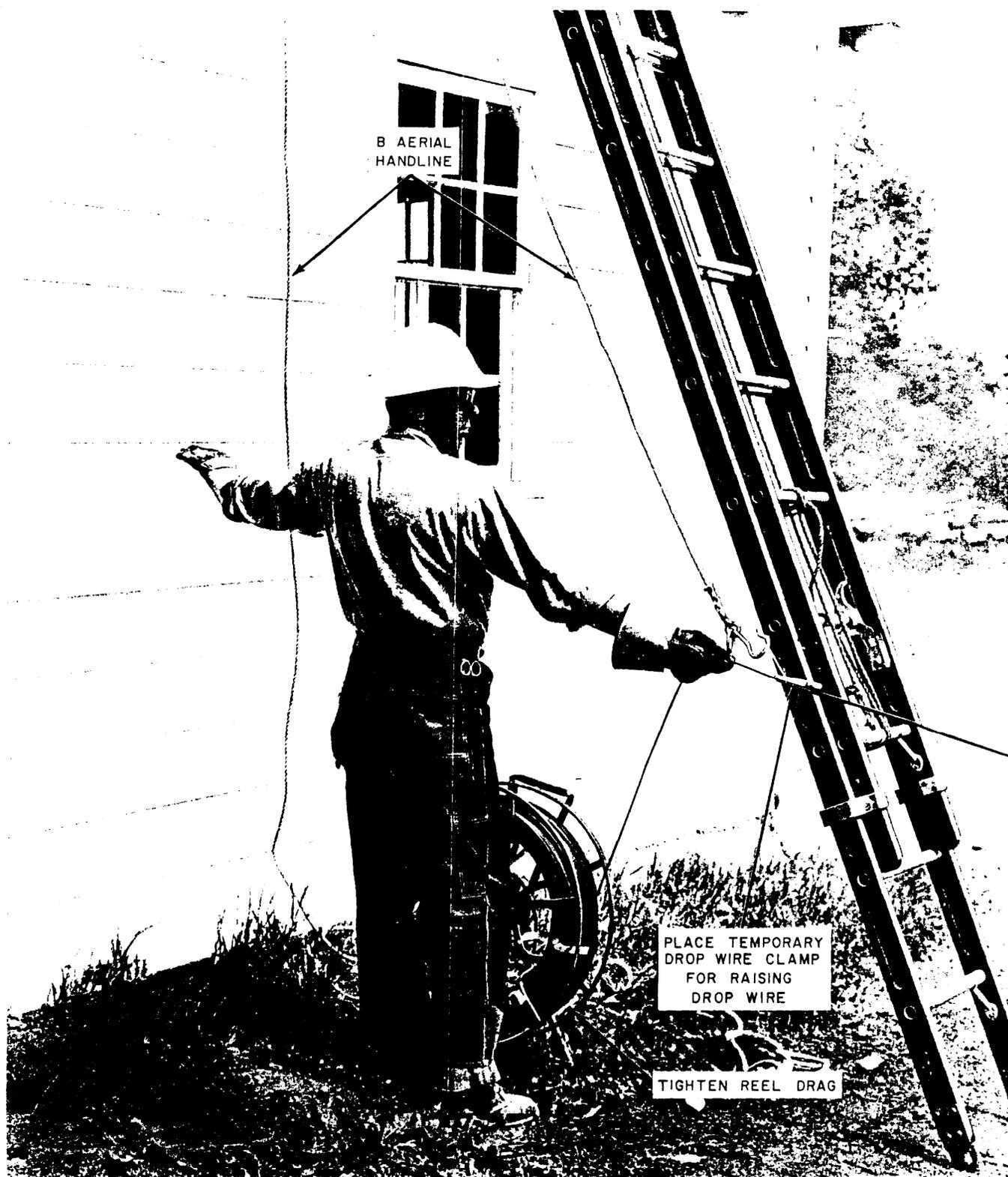
Fig. 31-Locating Temporary Drop Wire Clamp
