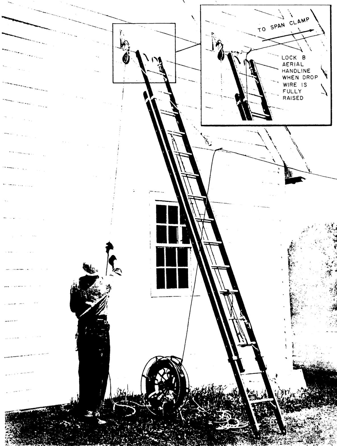
Fig. 32-Raising Drop Wire to Building Attachment
