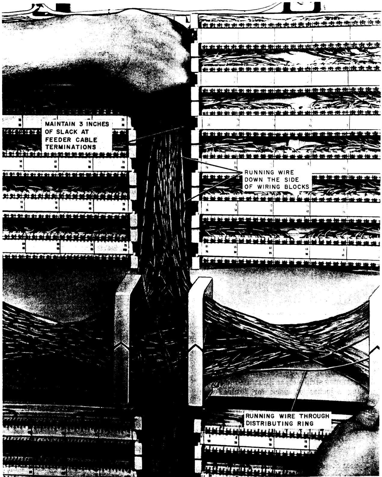
Fig. 4—Positioning Cross-Connecting Wire
