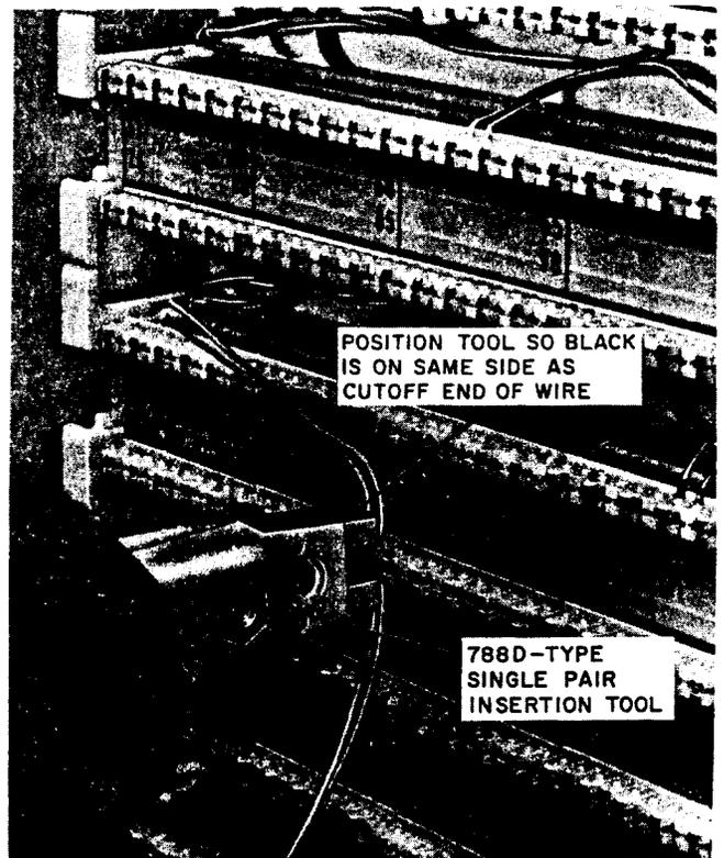
Fig. 3—Seating and Cutting Cross-Connecting Wire Into Connecting Block
