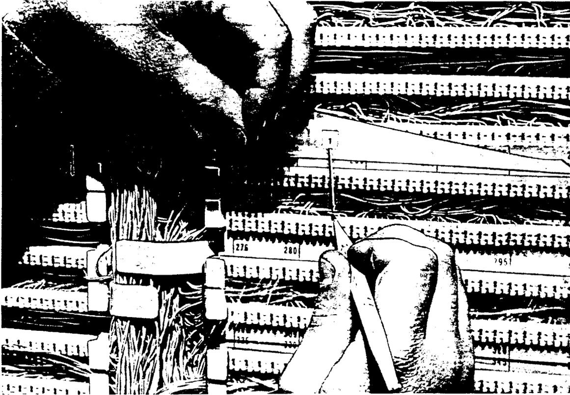
Figure 24. Removing Insulation from Block
