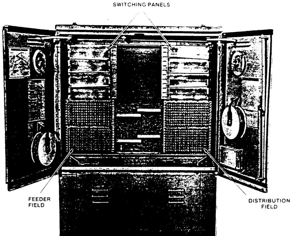
Figure 6. Method of Pair Identification—RAI-A—Two Panels
