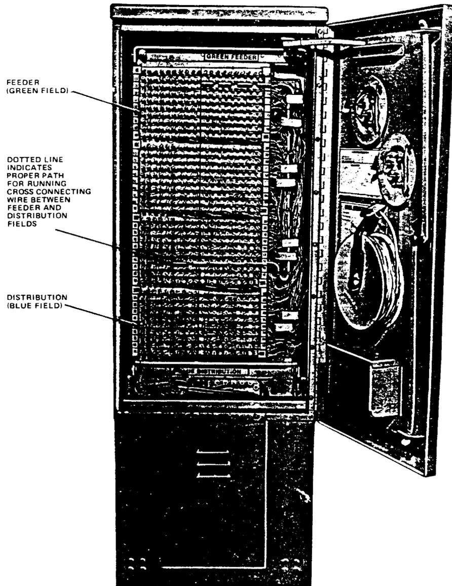
Figure 2. Method of Pair Identification—40-Type Cabinet Equipped with One Panel of 76-Type Binding Post
