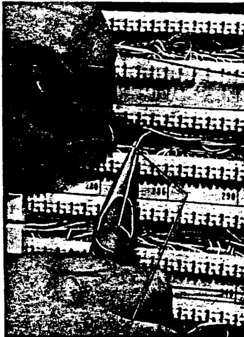
REMOVING CROSS-CONNECTING WIRES
