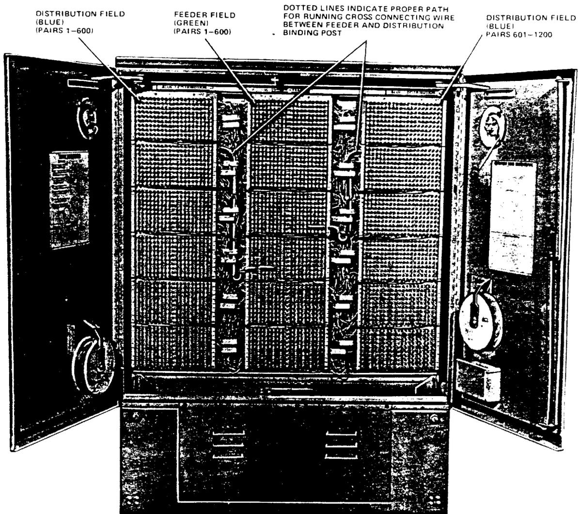
Figure 3. Method of Pair Identification—40-Type Cabinet Equipped with Three Panels of 76-Type Binding Post
