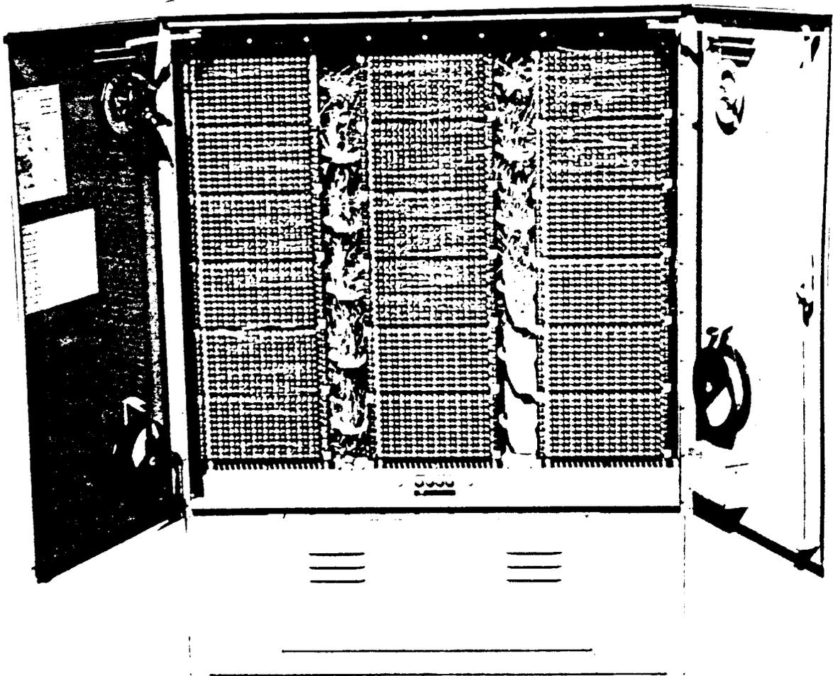
**Figure 4. Method of Pair Identification—40-Type Cabinet Equipped with Three Panels of 99-Type Connecting Blocks**
