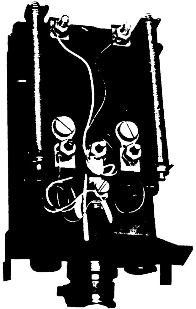
**Figure 42—106C Protector (LA) in C Customer Service Closure With Buried Service Wire**
