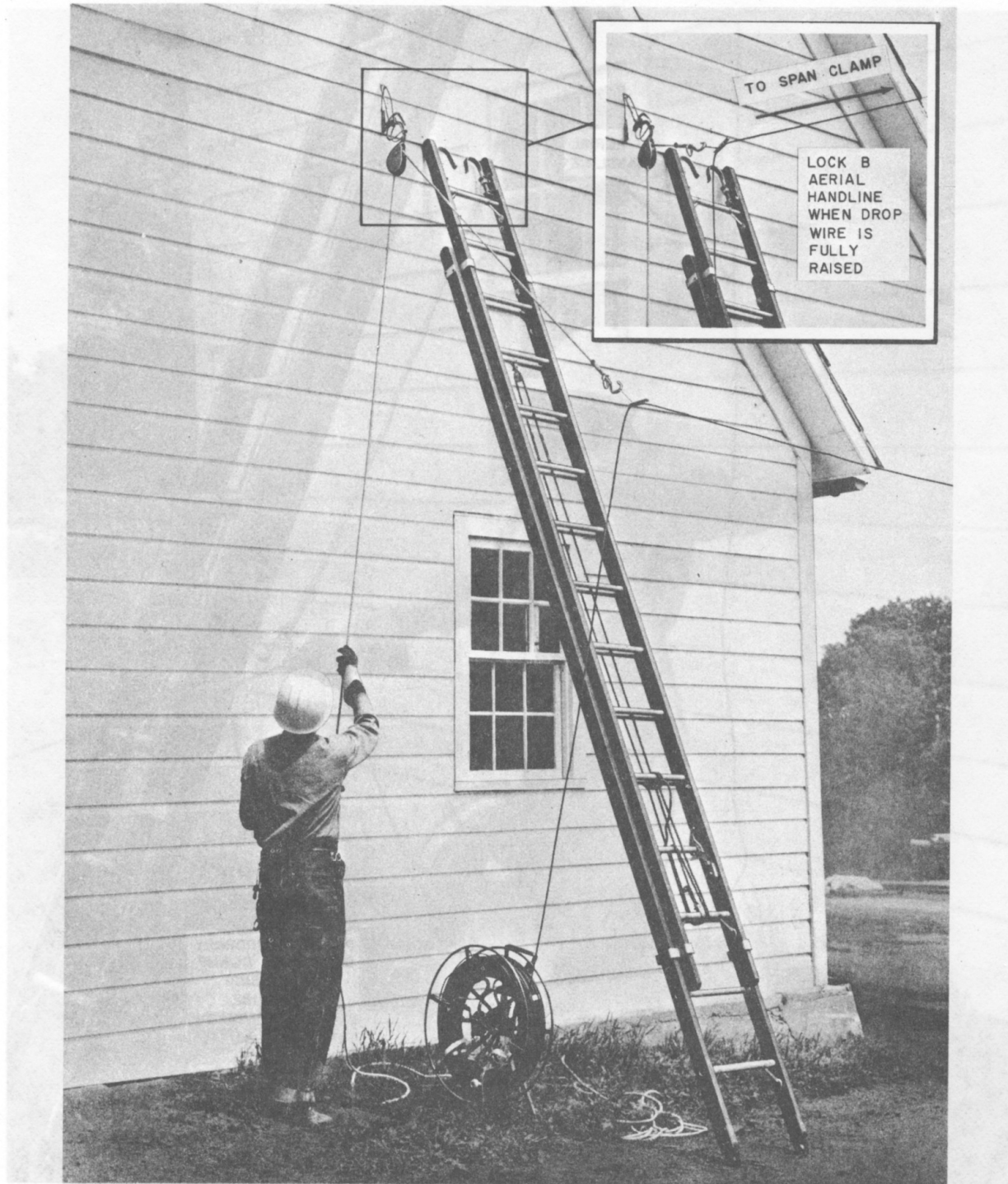
Fig. 9—Raising Drop Wire to Building Attachment
