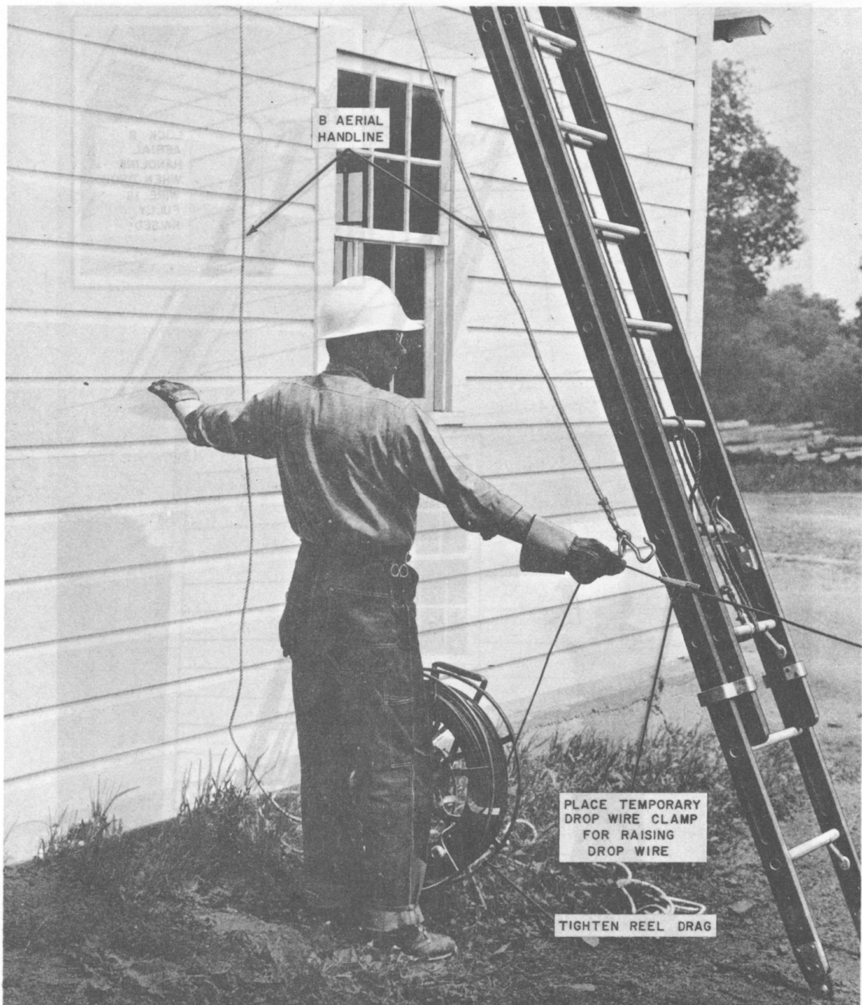
Fig. 8—Locating Temporary Drop Wire Clamp
