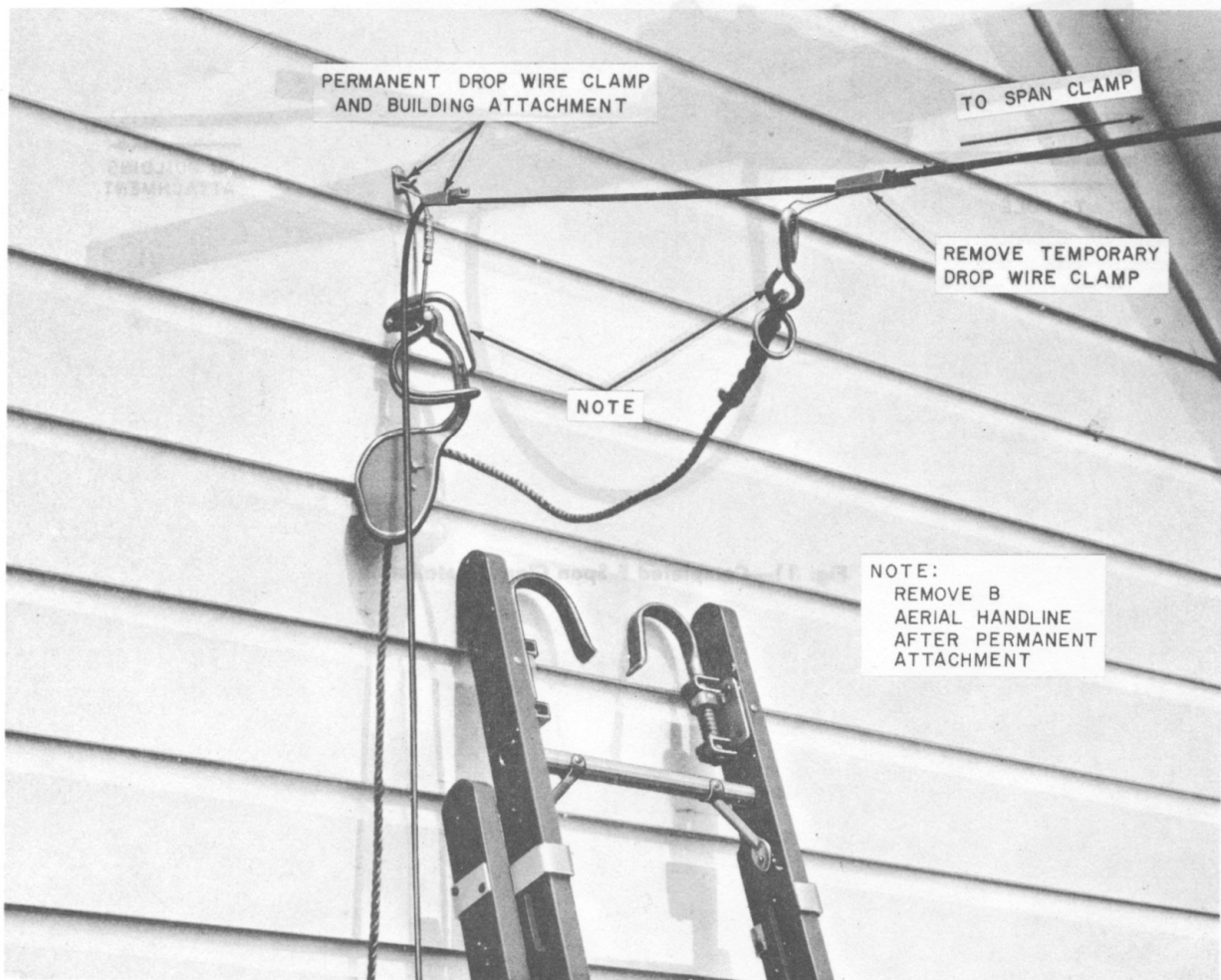
Fig. 10—Completing Permanent Building Attachment
