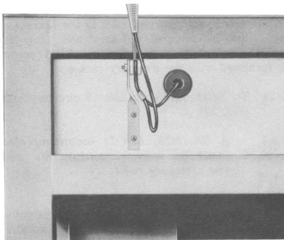
◆Fig. 13—Corner Bracket for First Attachment◆
