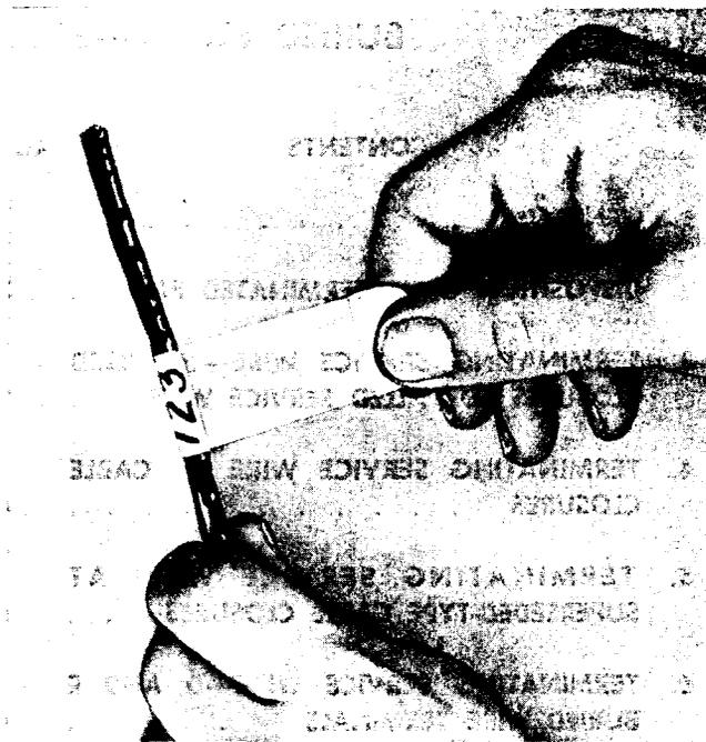
Fig. 1—♦Placing Self-Laminating Label♦
