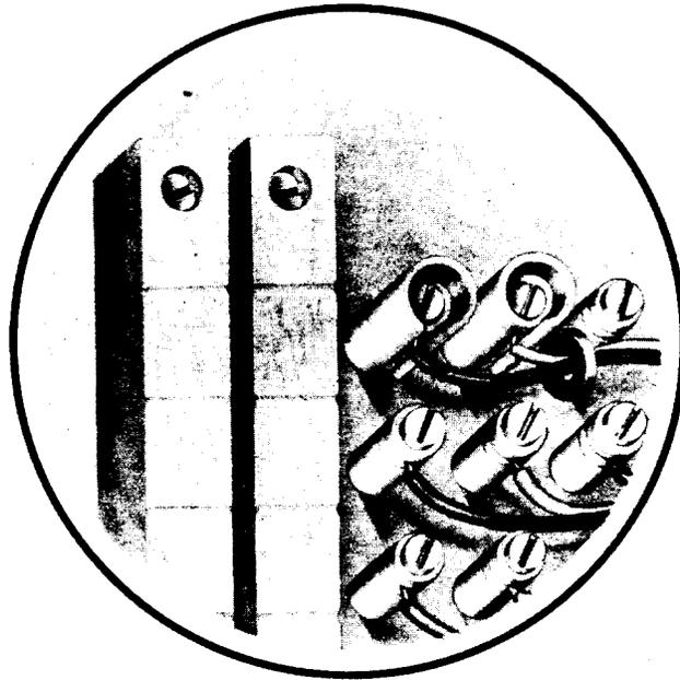
Figure 27 - Binding Post Insulators Installed at BD-Type Cable Terminals
