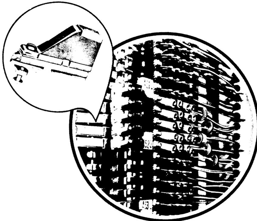
Figure 32 - SSP on Frame Equipped with 444A Test Jacks on 401 Connector
