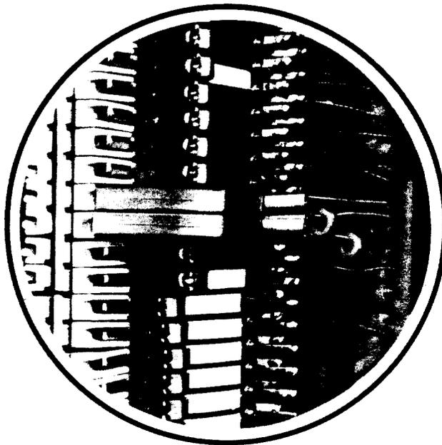
Figure 30 - KS-14539, L5 Guard Installed on 1177 Protector
