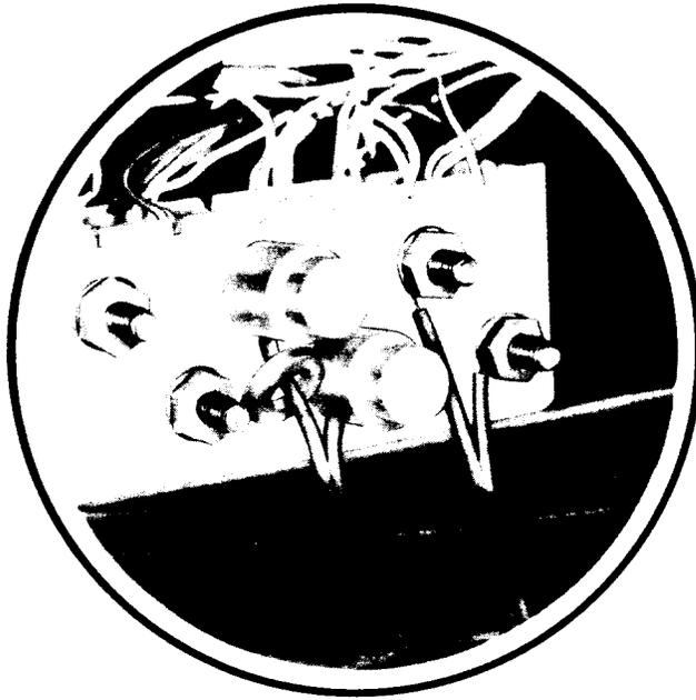
**Figure 25** - E Binding Post Caps and Indicators Installed on 49A Cable Terminals
