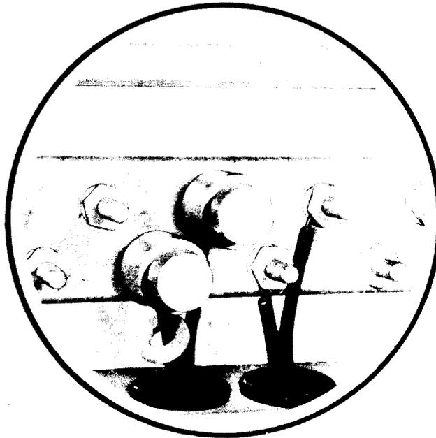
Figure 20 - Installed Binding Post Caps and Indicator at N-Type Cable Terminals
