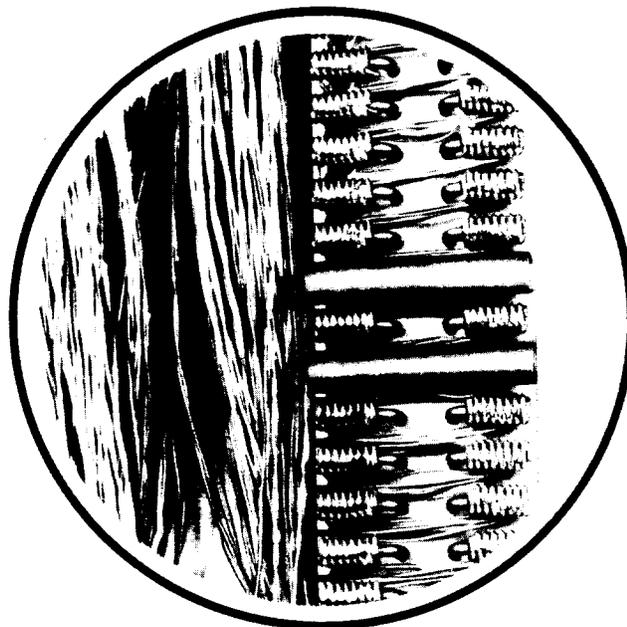
**Figure 23** - B Coil Spring Insulators (MD) Installed on 70-type Connecting Block (MD)
