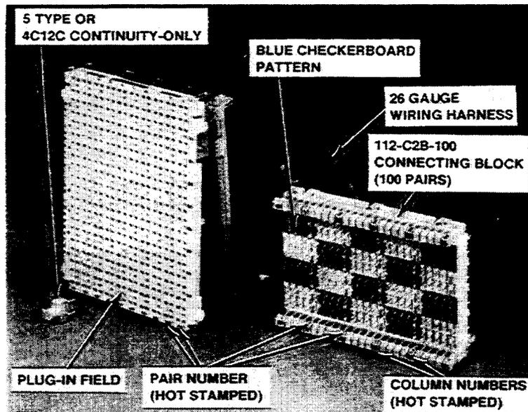
**Figure 2. 407D1-100 Connector — Front View**
