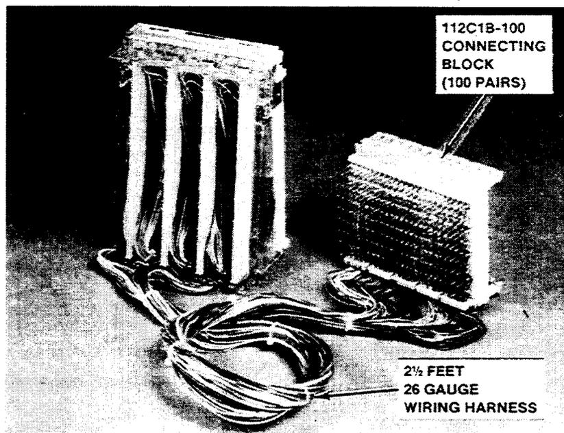
Figure 5. 407F1-100 Connector — Back View
