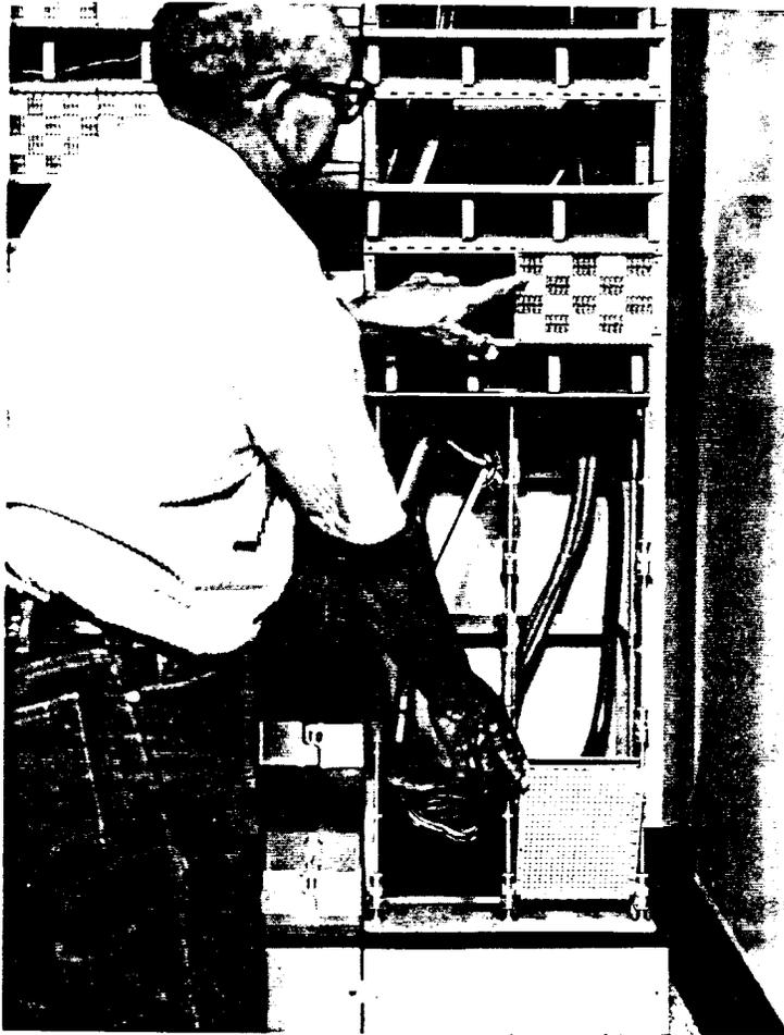
Figure 22. Routing UL Connector Stub Cable on Mini *COSMIC* Frame (Front View)
