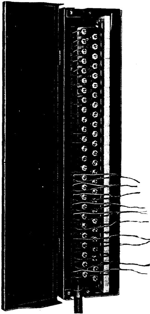
Fig. 8—Terminating Inside Wiring Cable
