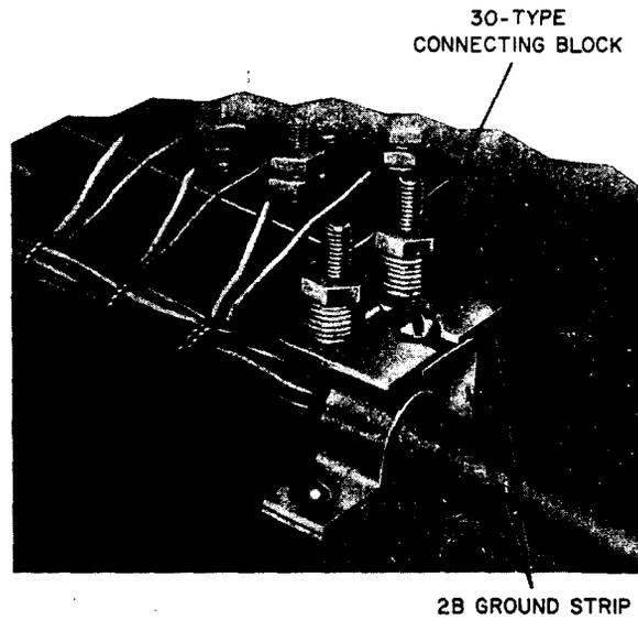
**Fig. 5—Installation of 2B Ground Strip**
