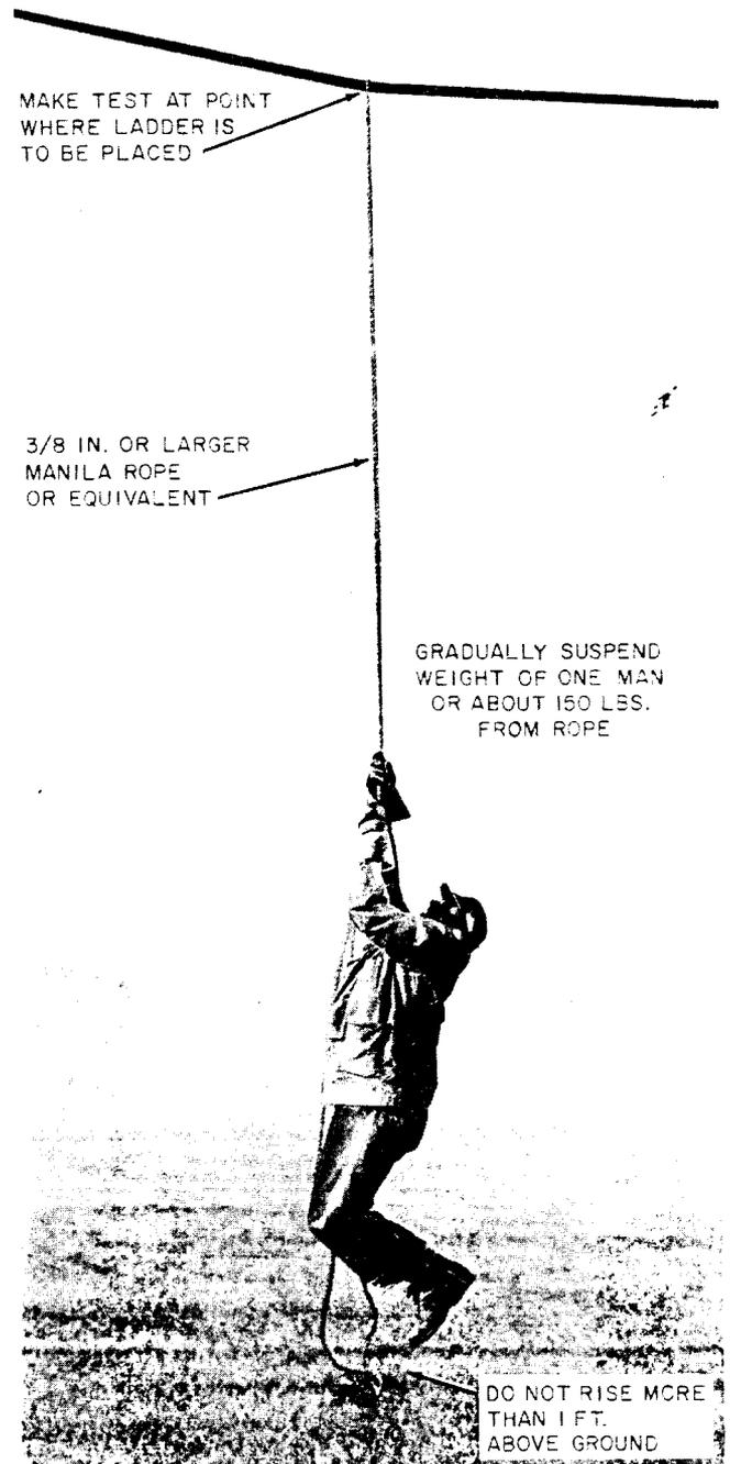
**Fig. 2—Testing Strand Prior to Placing Ladder**
