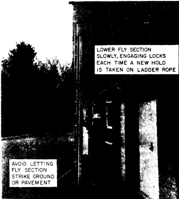
Fig. 22—Fly Section Lowered
