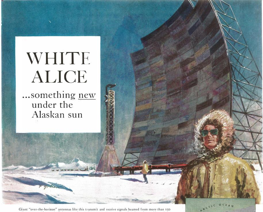
Giant "over-the-horizon" antennas like this transmit and receive signals beamed from more than 150 miles away and bounced off the troposphere, a layer of air five to seven niles above the earth's surface.
