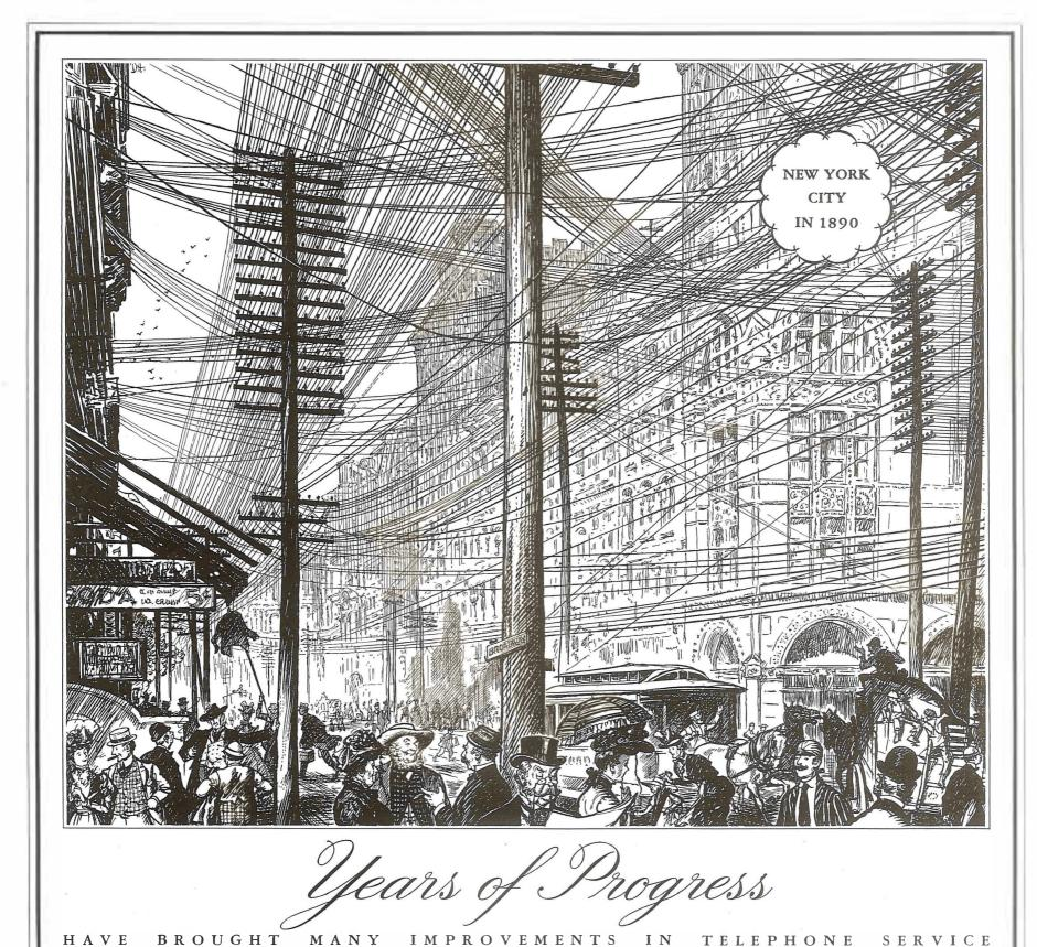
BACK in the early days of the telephone, practically all wires were carried overhead on poles or on house-tops. Some of the tallest poles carried as many as thirty crossarms and three hundred wires.
