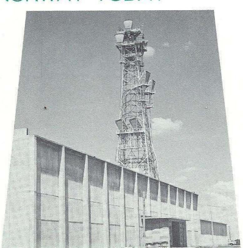
During 1961 an additional 138,000 square feet added for new 4A switching center. From an original structure of 803 square feet, the repeater station has mushroomed to 153,000 square, feet, increasing its size 193 times. Only eight-legged radio relay tower in Bell System, 242-foot tower supports 16 antennas serving eight radio directions.
