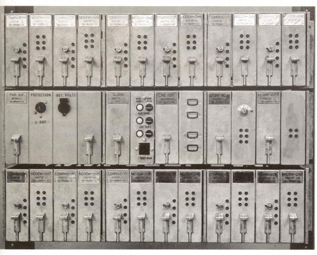
Plug-in N2 units mounted in three die-cast 23" aluminum shelves provide twelve-channel carrier transmission. An 11' 6" bay holds eight of these terminal arrangements, giving a total of 96 carrier circuits. A 9' bay provides 72 circuits.
