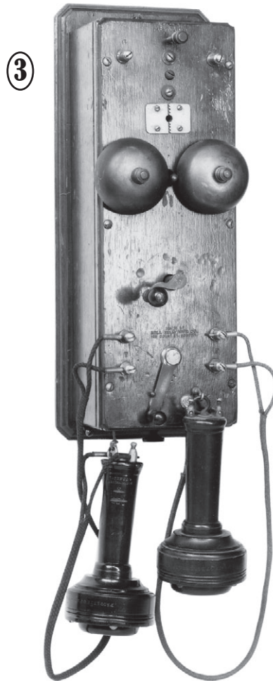
Figure 3: Williams' coffin telephone of 1878 with Bell's butter-stamp telephones and Watson's ringer.
