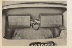
MOBILE TRANSMITTER AND RECEIVER — Final link in the equipment required is this transmitting unit, with about 20 watts power, and receiving set including selective signaling device. Shown here installed in the trunk of a passenger car, this equipment may be mounted inside a truck body or on the running board — wherever space permits.
