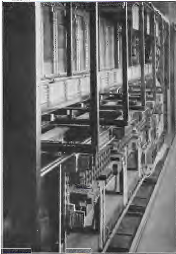
Rear View of No. 11 Multiple Switchboard.
