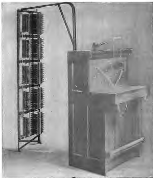
No. 1430 Type Main Distributing Frame
