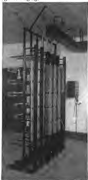
No. 1407C Testing Cabinet Connected to Main Distributing Frame
