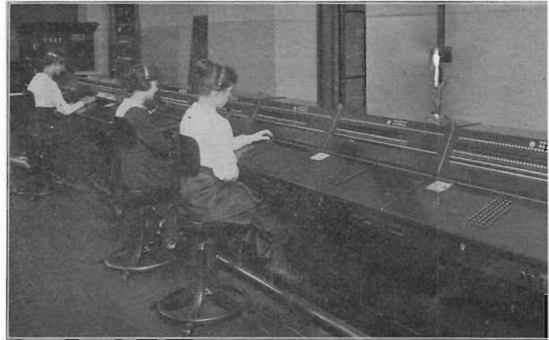
Figure 19. Typical installation of Cordless B positions in a machine switching office.
