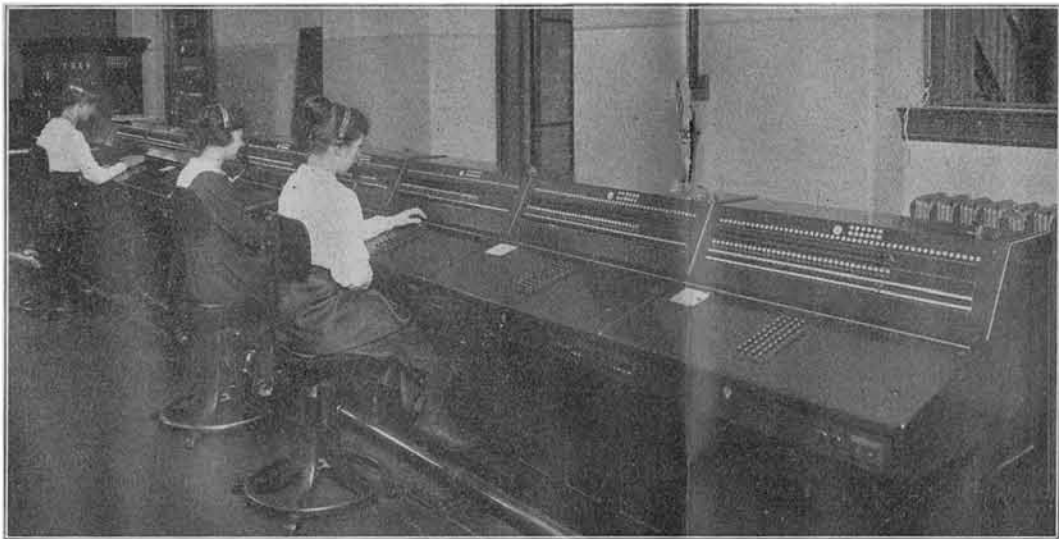
Figure 19. Typical installation of Cordless B positions in a machine switching office.
