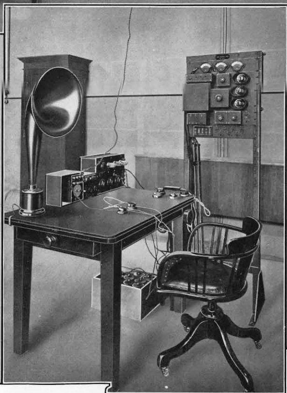
Control Room of typical Broadcasting Station, showing special Input Panel
