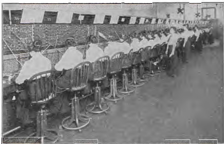
Central Battery Multiple Switchboard at Yonkers, N. Y.
