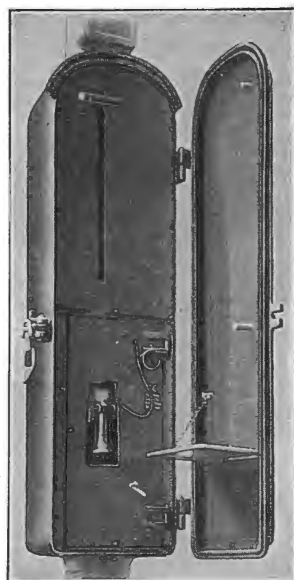
Selector Signal Mechanism, and Telephone Apparatus Case
