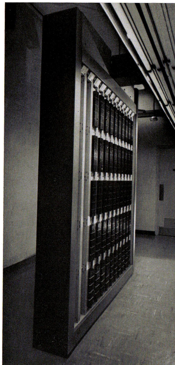
Central office equipment can be disconnected from the protector frame merely by pulling the protector forward to a detent position. This action disconnects only the central office equipment and not the outside cable pair which remains protected.
