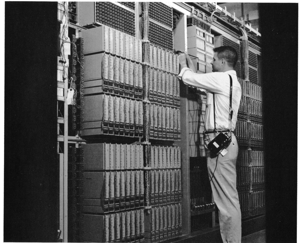
J. Bodirae, a Western Electric craftsman, performs an installation test on line switching frames.
