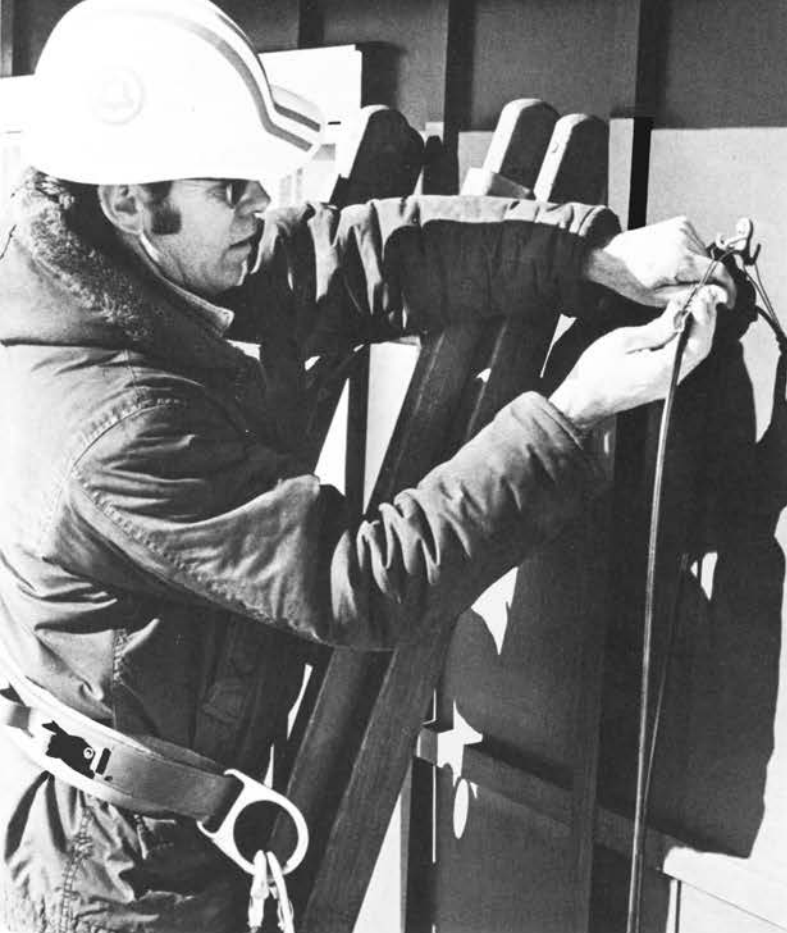
New drop wire insulated with polyvinyl chloride (PVC) makes the installation job easier. Here, at left, it is being used in a test installation by John Apgar of Bell Labs' Chester, New Jersey, location. The wire is 30 percent lighter than the wire it re-
