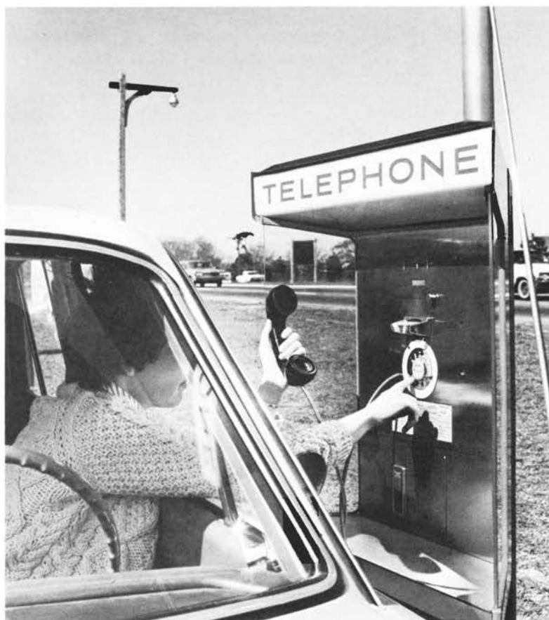
The walk-up drive-up enclosure offers easy accessibility in a variety of configurations. It can be used singly along highways like this enclosure on Long Island, New York, or it can be used as a single, double, or quadruple installation for walk-up use.
