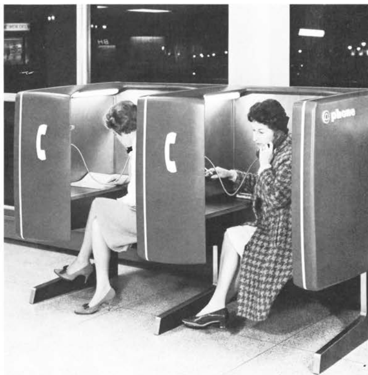
The low-profile enclosure, an experimental design, is intended for airports, civic centers, and other deluxe applications. Low-profile booths can be assembled in groups, in-line or back-to-back.
