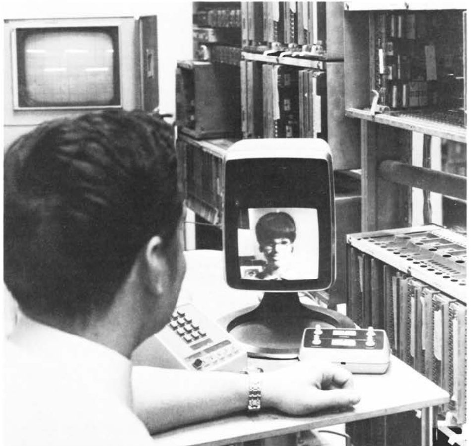
F. J. Bogart of Bell Labs 850A PBX Group at Denver, Colo., tests the conferencing capabilities of a new call switching machine for PICTUREPHONE® service. The 850A private branch exchange will handle up to 89 Picturephone lines per business customer location. The PBX also may be used for Picturephone intercom networks.
