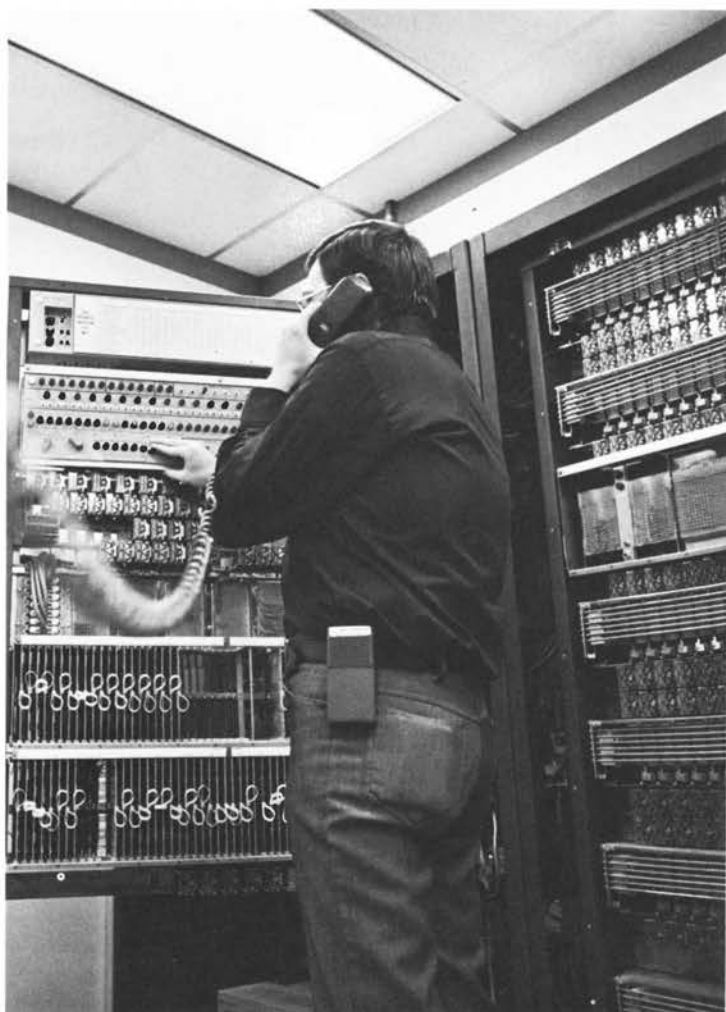
Maintenance panel. Larry A. Hendren, Communications Serviceman from Mountain Bell, monitors a test call being processed by an 812A PBX installed at Bell Labs' Denver location. This panel helps a craftsman locate problems quickly and efficiently.
